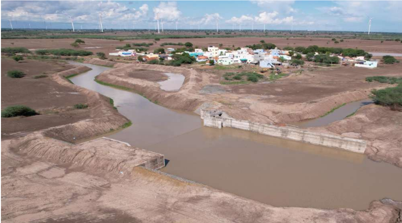
Thoothukudi District - Ottapidaram Taluk - Mullur Muthukumarapuram Village - Construction of new Regulator across Malattar Odai - Estimate amount :Rs.425.11 Lakh
