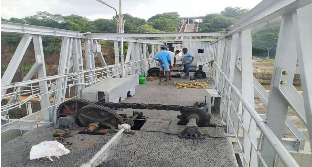
Cuddalore District - Chinnasalem Taluk - Vadakananthal Village- Replacement, Fabrication and Erection of Vertical Shutter in Old Existing Spillway vent 1 & 2 with hoisting arrangements in Gomukhi Dam– Estimate Amount :Rs.12.40 Crore
