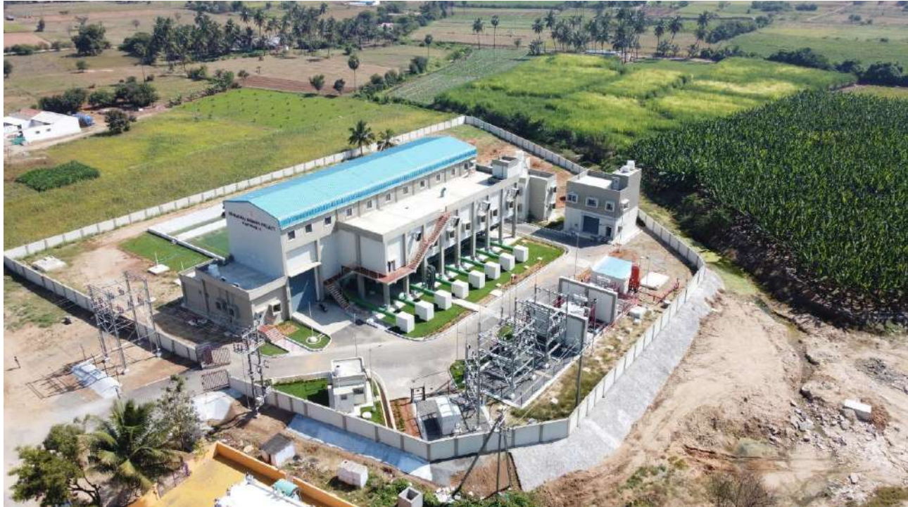
Erode District - Nambiyur Taluk - Athikadavu Avinashi Pumping Scheme, Pumping station V- Emmampoondi Village - Estimate Amount Rs.1916.417 Crore
