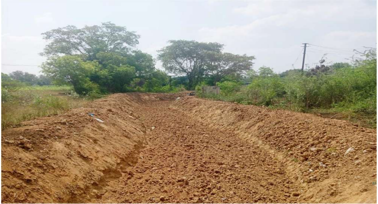
Villupuram District - Tiruvannainallur Taluk – Rehabilitation of Amoor Channel Estimate Amount:Rs.5.0 Crore
