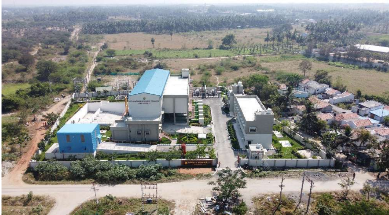
Coimbatore District - Annur Taluk - Athikadavu Avinashi Pumping Scheme, Pumping station VI - Annur Village - Estimate Amount Rs.1916.417 Crore
