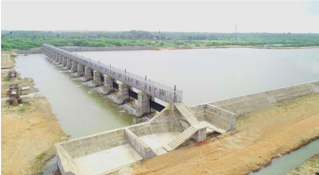
Villupuram District - Marakanam Taluk - Reclaiming Kazhuveli Tank for storage of fresh water and sea water intrusion control measures and recharge shaft Well/ Shafts – Estimate Amount : 166.75 Crore
