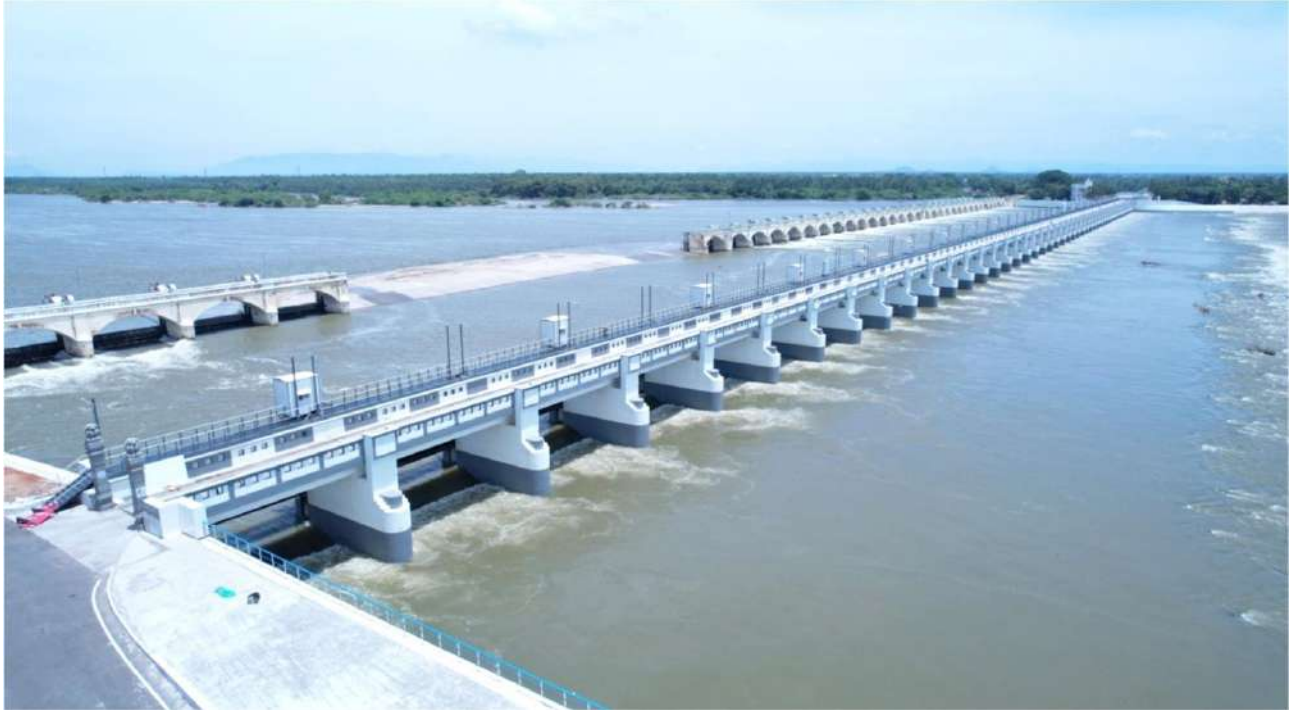
Tiruchirapalli District – Vathalai Village (Upper Anicut– Mukkombu) – New Regulator across Kollidam River- Estimate Amount Rs. 414.00 crore
