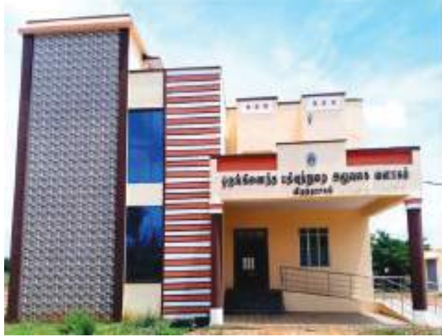
New Integrated Registration Complex Building of Vridachalam Registration District.
