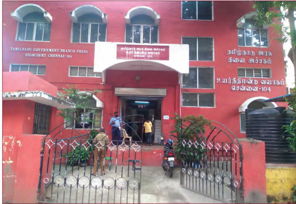
Government Branch Press, Madras Highcourt campus, Chennai.
