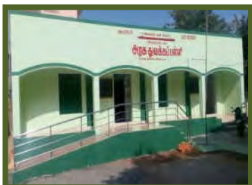
Picture 36 - Additional Classroom building
