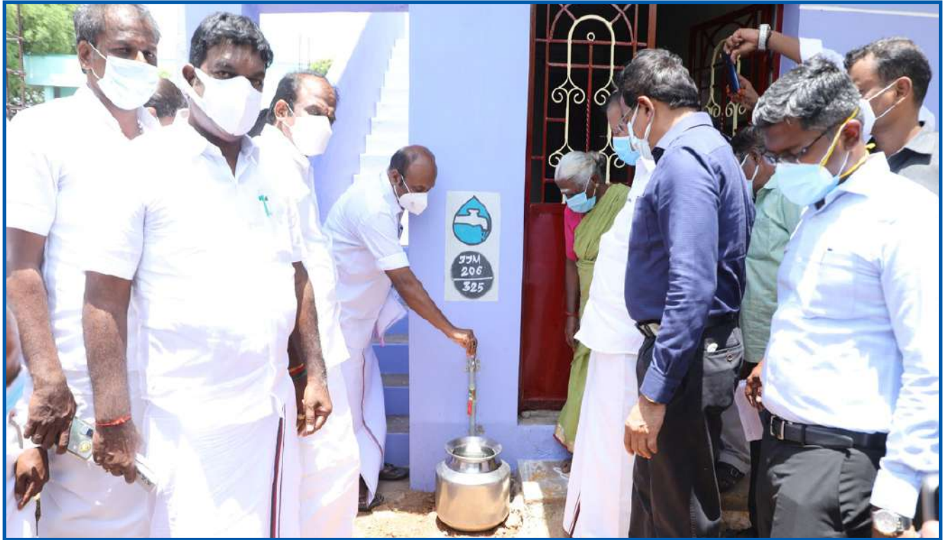
Household water supply connection under Jal Jeevan Mission
