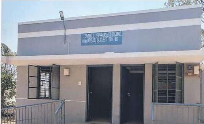
Office cum Residential Firka Quarter – Krishnagiri District, Sulagiri Taluk, Sulagiri Firka
