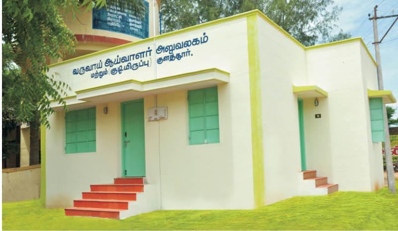
Revenue Inspector's Office-cum-Quarters, Kulathur, Thoothukudi District.
