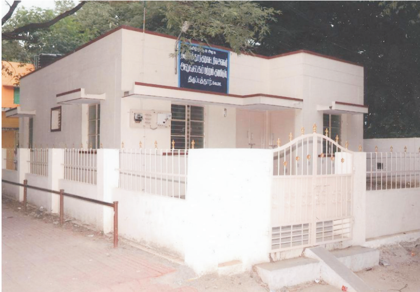
Firka Surveyor Office-cum-Quarters, Tirupathur, Vellore District.
