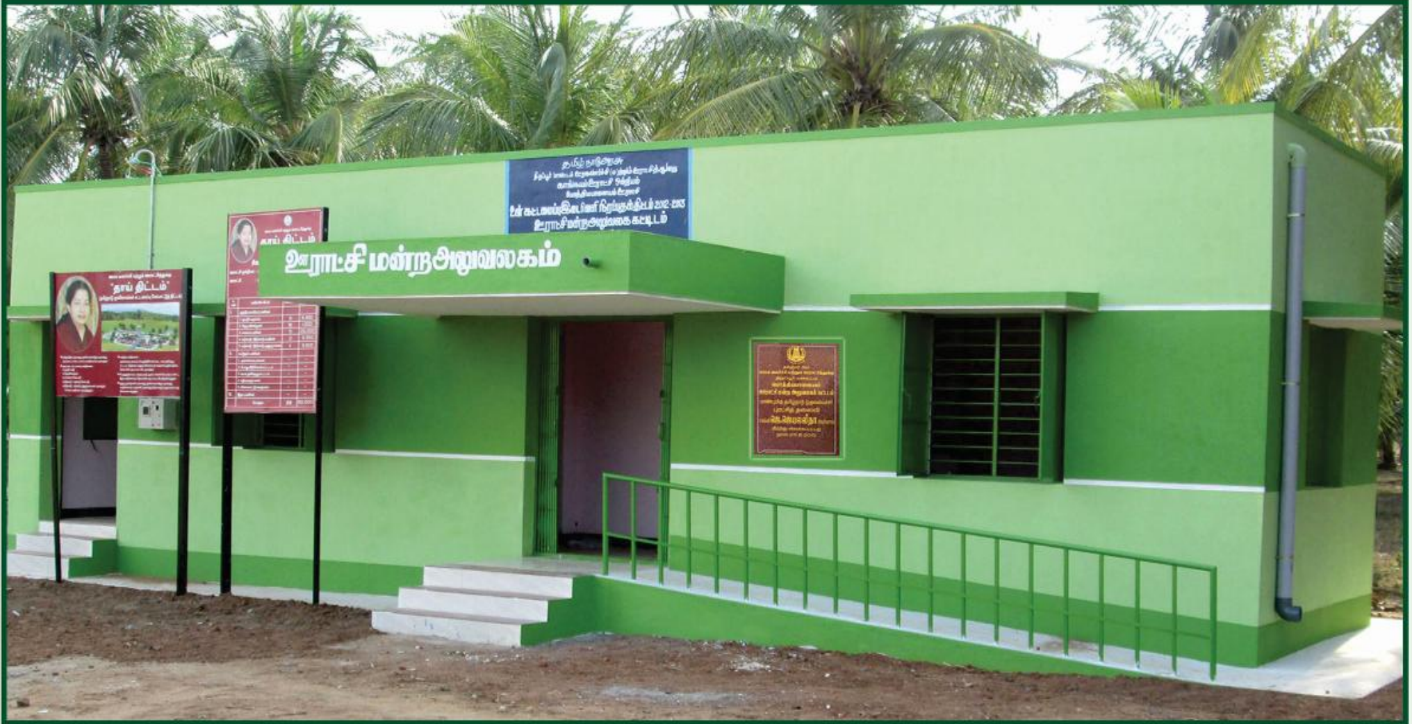
New Village Panchayat Office
