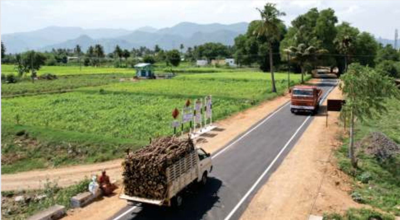
Rural Road MRL 21 SU – Manivizhuthan Pudur via Manivizhuthan North Pudur (1/600-5/900 km) laid under Pradhan Mantri Gram Sadak Yojana (PMGSY-III) in Thalaivasal Panchayat Union of Salem District, at an estimate of Rs.232.30 Lakhs
