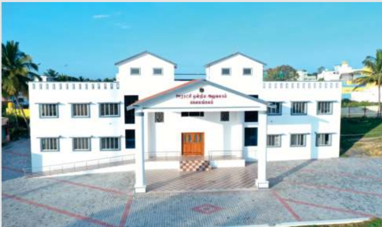
Panchayat Union Office Building constructed at Kelamangalam of Krishnagiri District under Scheme component of Pooled Assigned Revenue at an estimate of Rs.3.10 crore.
