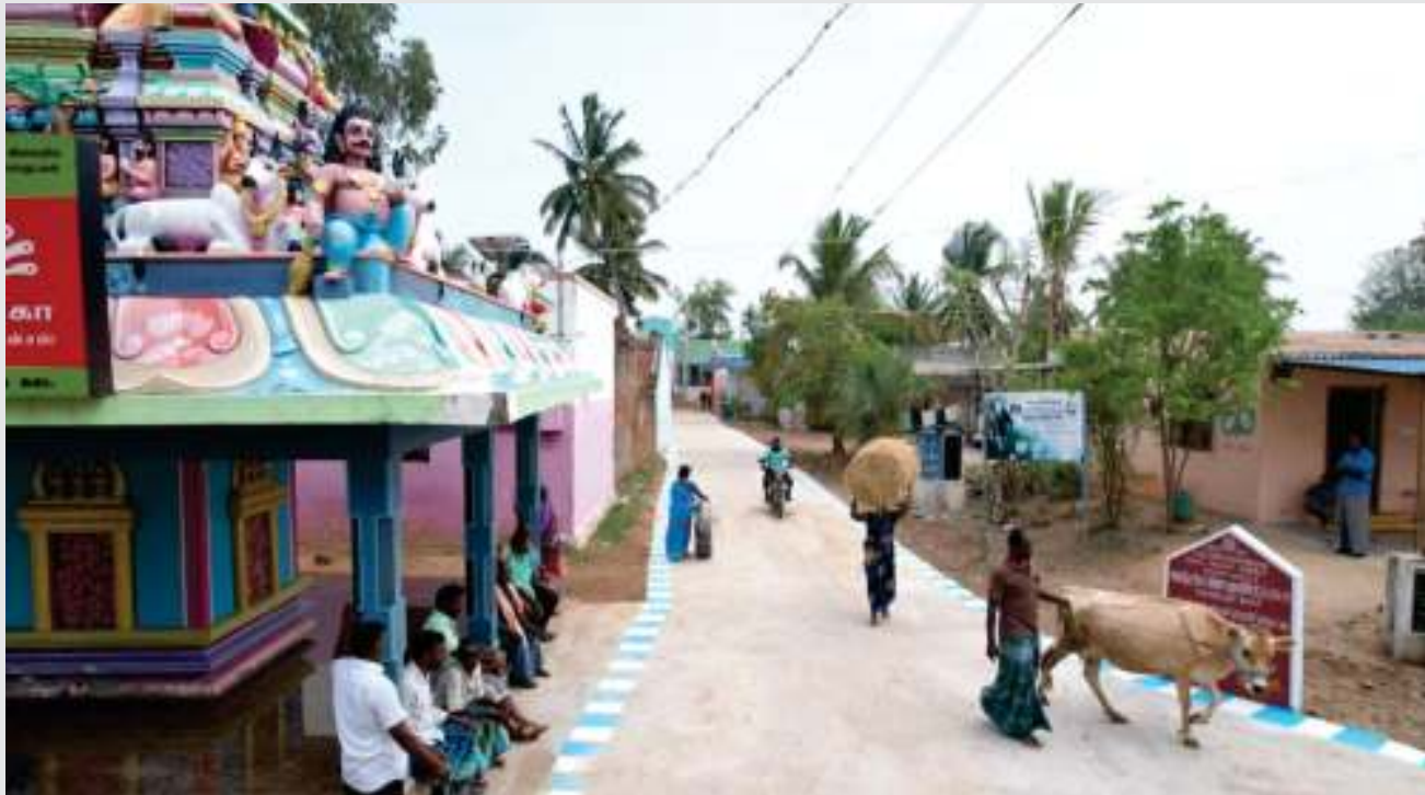
Cement road laid in Chinnapudur Vinayagar Koil Street under Anaithu Grama Anna Marumalarchi Thittam II at an estimate of Rs. 4.06 Lakhs in Semmandakuppam Panchayat, Dharmapuri Panchayat Union of Dharmapuri District
