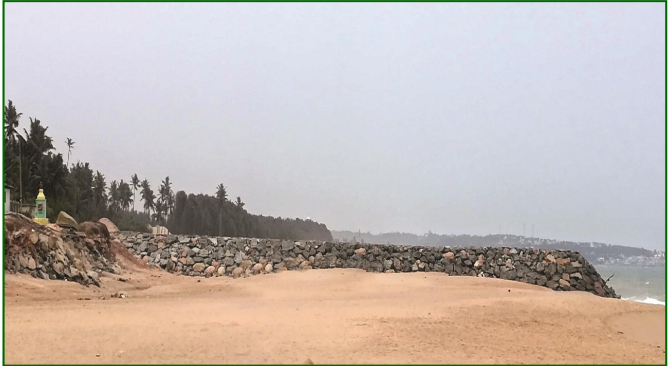
Kanniyakumari District – Groyne constructed in Mandakadu Puthoor (Estimate Amount Rs.7.82 crore)
