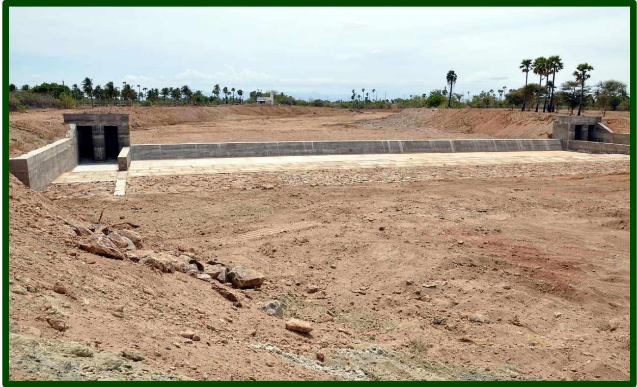
Karur District - Checkdam constructed across Nanganjiyar River in Sellivalasu Village
