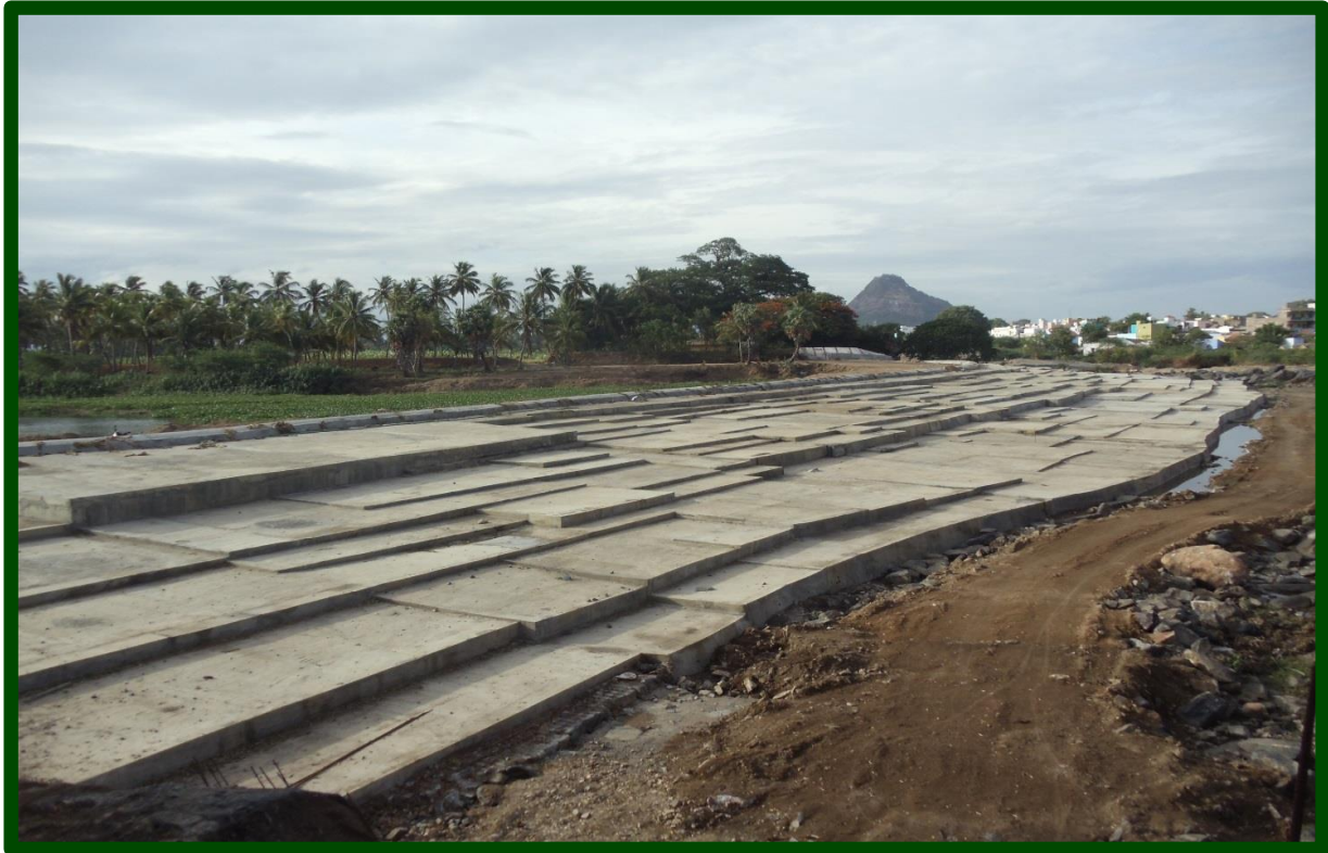
Erode District - Rehabilitated Kalingarayan Anicut across Bhavani River in Anainasuvampalayam Village
