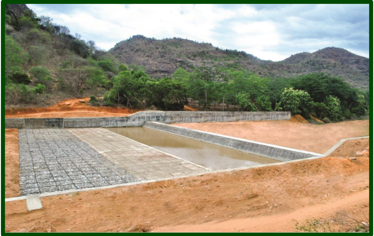
Theni District - Check dam constructed across Vaigai River in Valipparai Village
