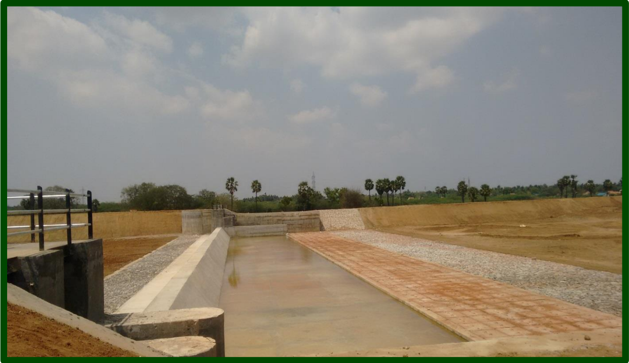
Sivaganagai District - Anicut Constructed across Manimuthar River in Udhayachi Village
