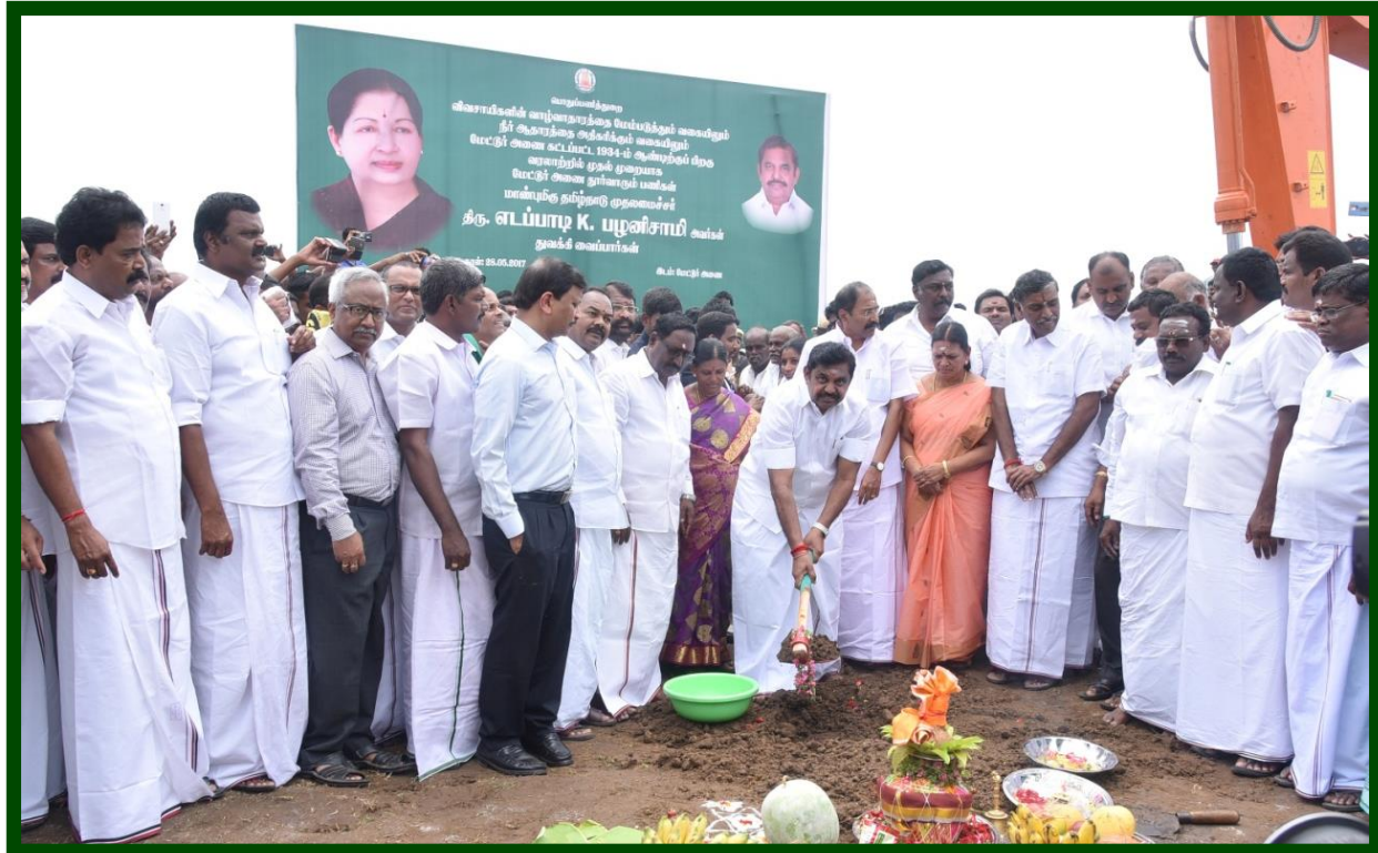
The Hon'ble Chief Minister inaugurated the Desilting Works in Mettur Dam of Salem District on 28.05.2017
