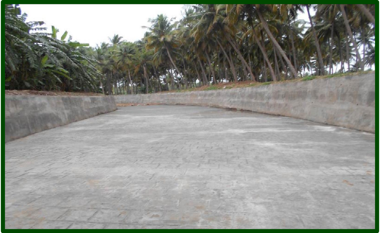
Theni District – Modernized Gullapuram Supply Channel in Gullapuram Village
