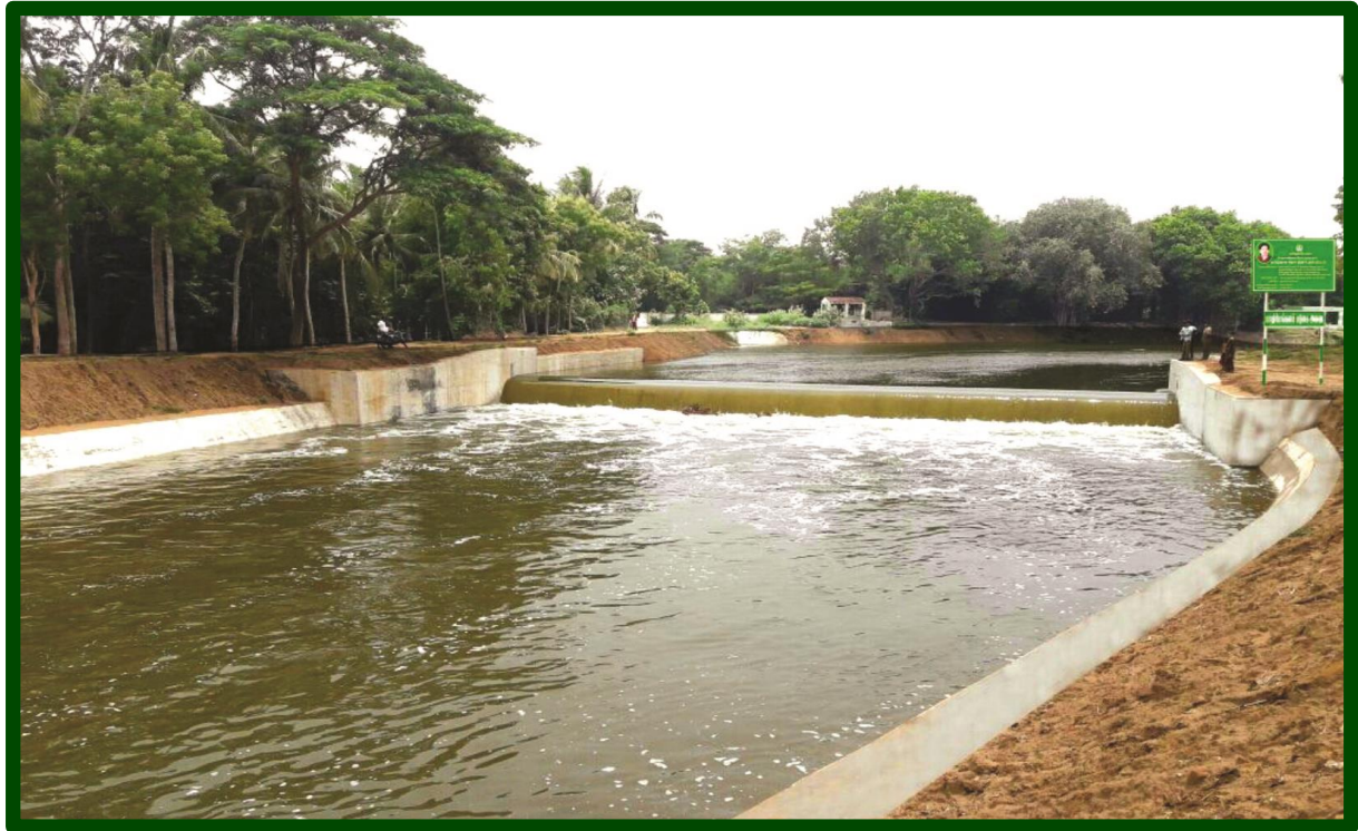
Nagapattinam District - Grade wall constructed across Cauvery River at L.S. 115.070 km to feed Kuthalam Channel in Mathirimangalam Village
