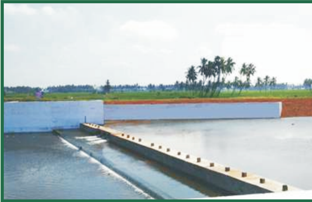
Rehabilitated Punganur Anicut across Ariyar River in Srirangam Taluk of Trichy District under NABARD Scheme
