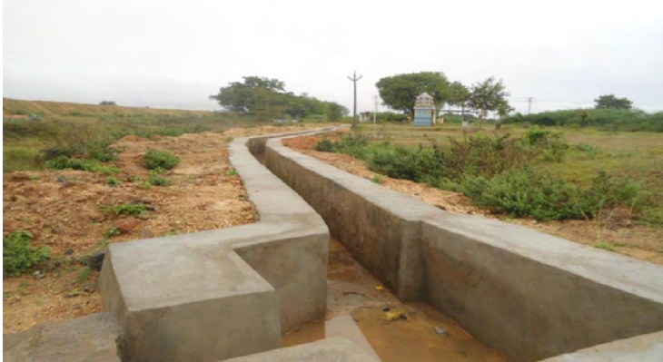
Lining of Field Channel
