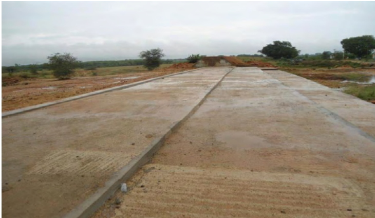
Rehabilitation of Surplus weir
