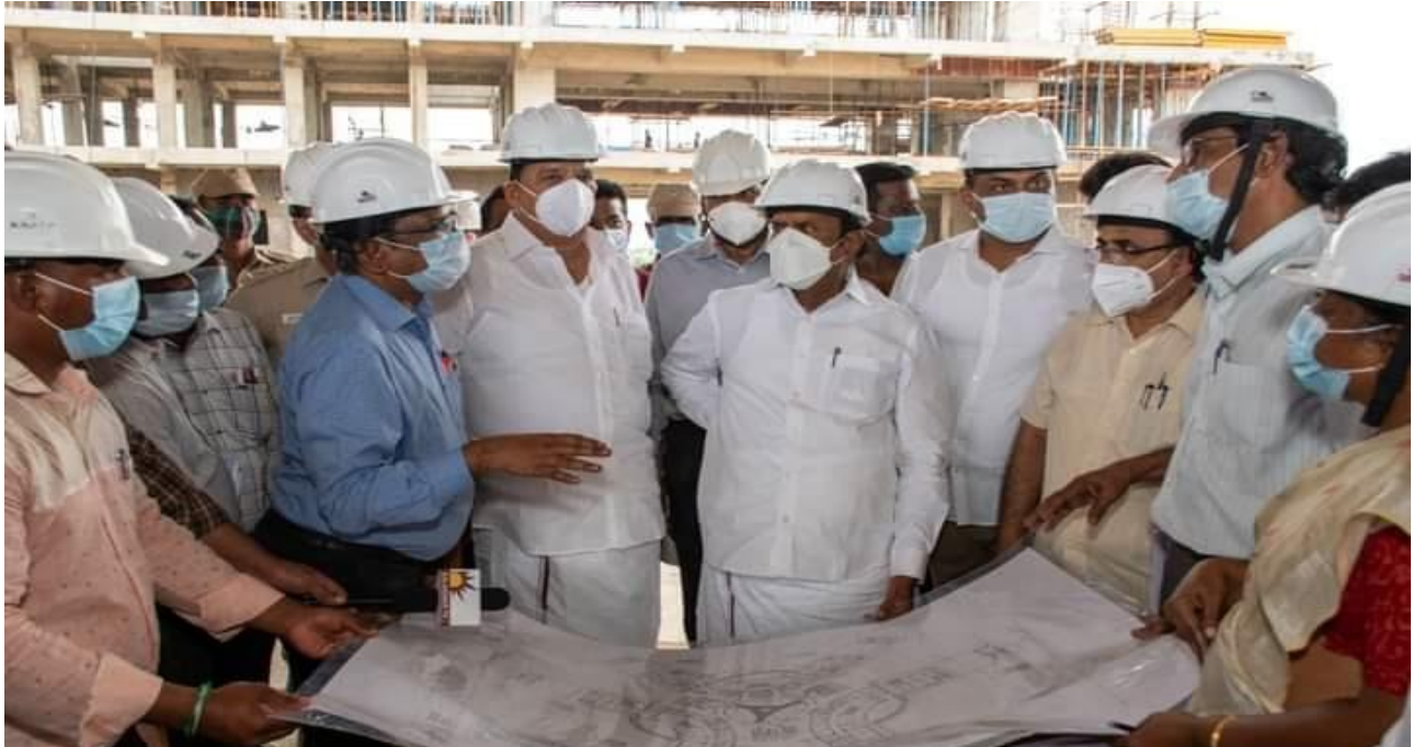
Inspection of the work progress at Ranipet Collectorate Building by Hon'ble Minister for Public Works along with Hon'ble Minister for Handlooms and Textiles on 14.07.2021
