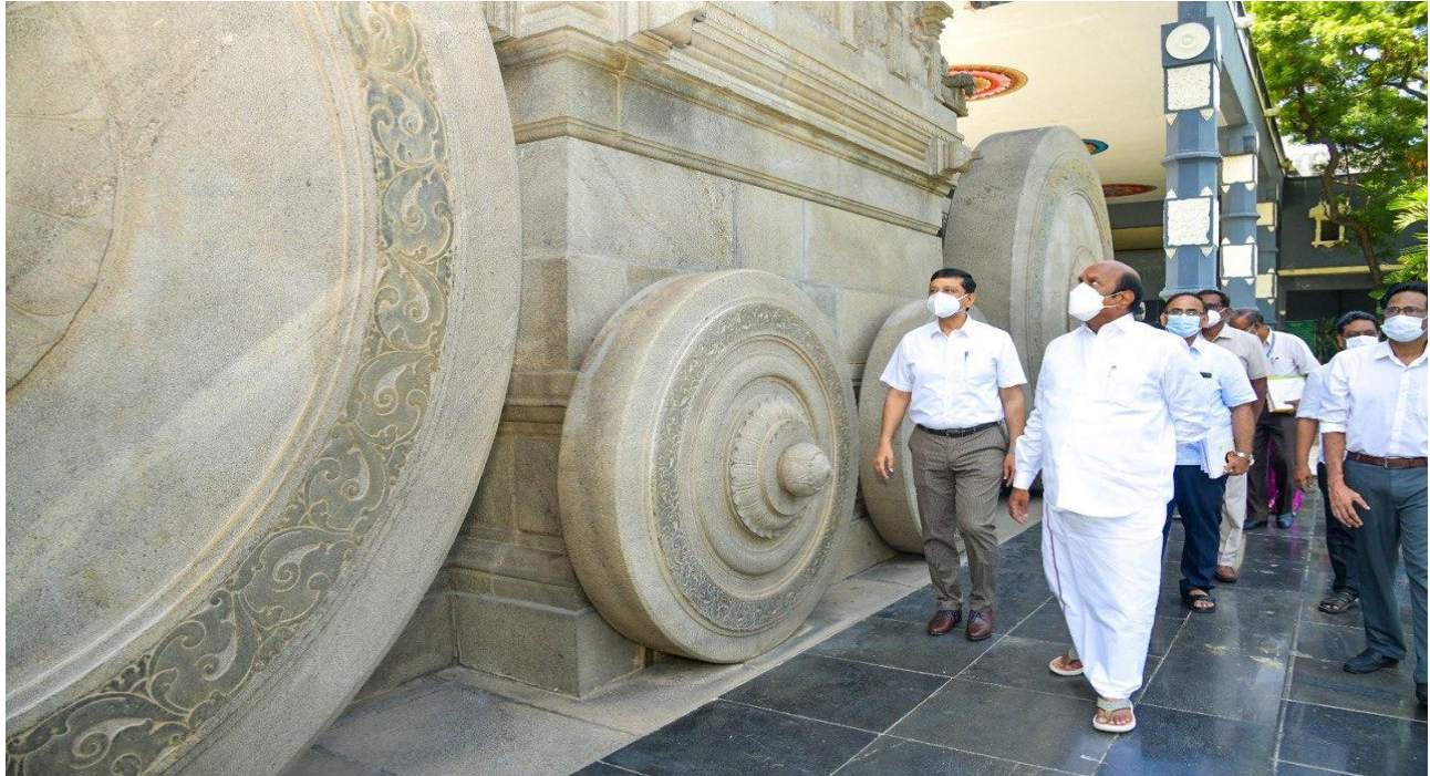
Hon'ble Minister for Public Works inspected the Valluvar Kottam at Chennai on 02.07.2021 for carrying out renovation work
