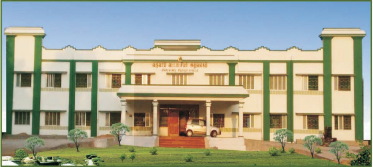
Taluk Office Building at Vikkiravandi in Villupuram District
