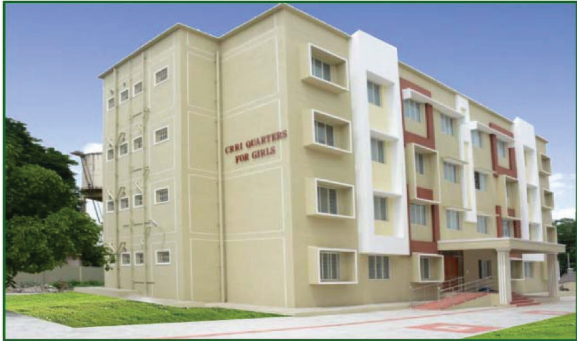
CRRI Quarters for Boys and Girls in Government Mohan Kumaramangalam Medical College at Salem in Salem District
