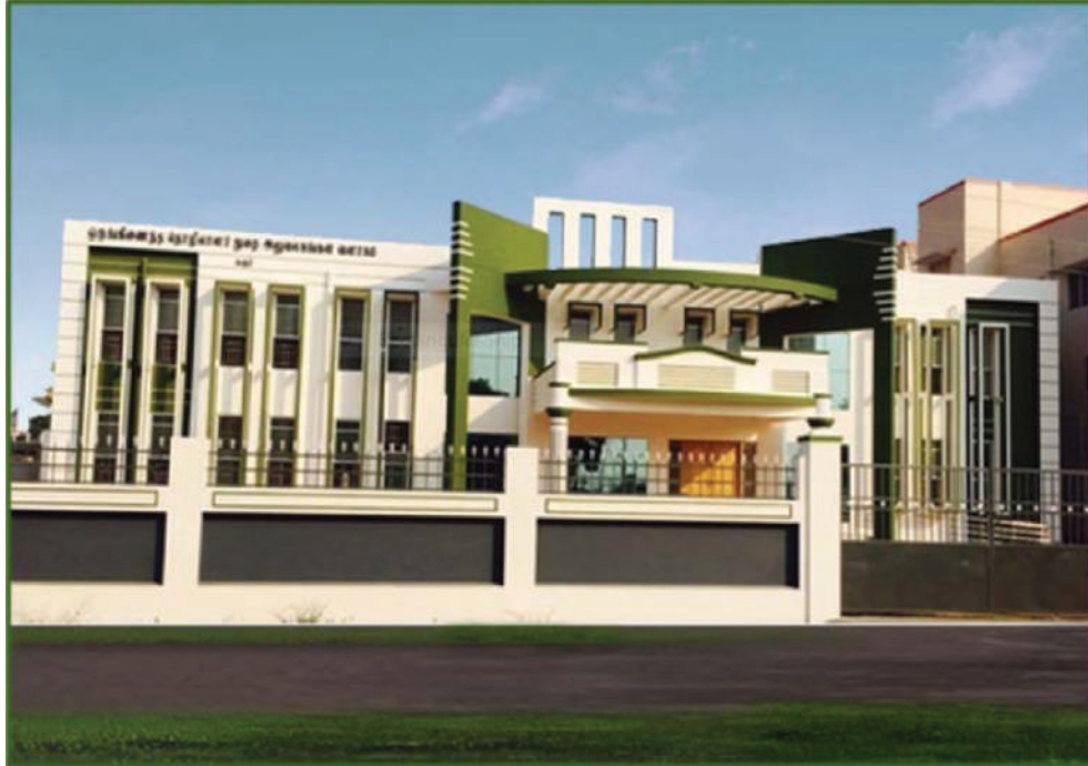
Integrated Office Complex Building for Labour Department at Karur in Karur District
