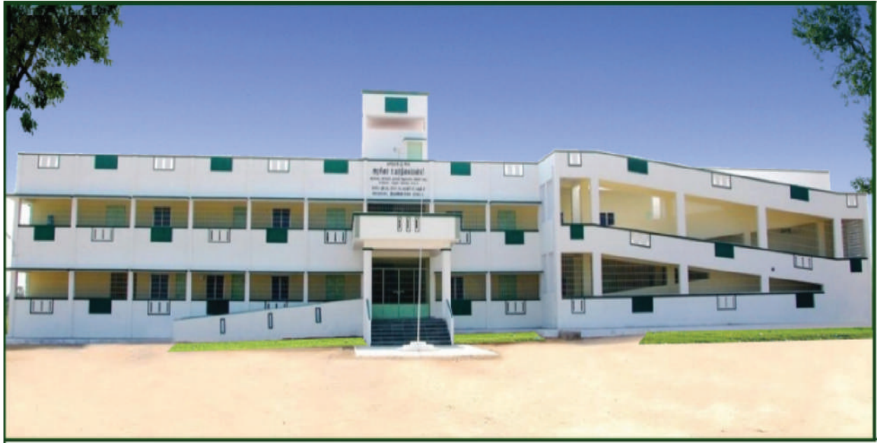
Government High School Building at Kodiylam in Tiruvannamalai District
