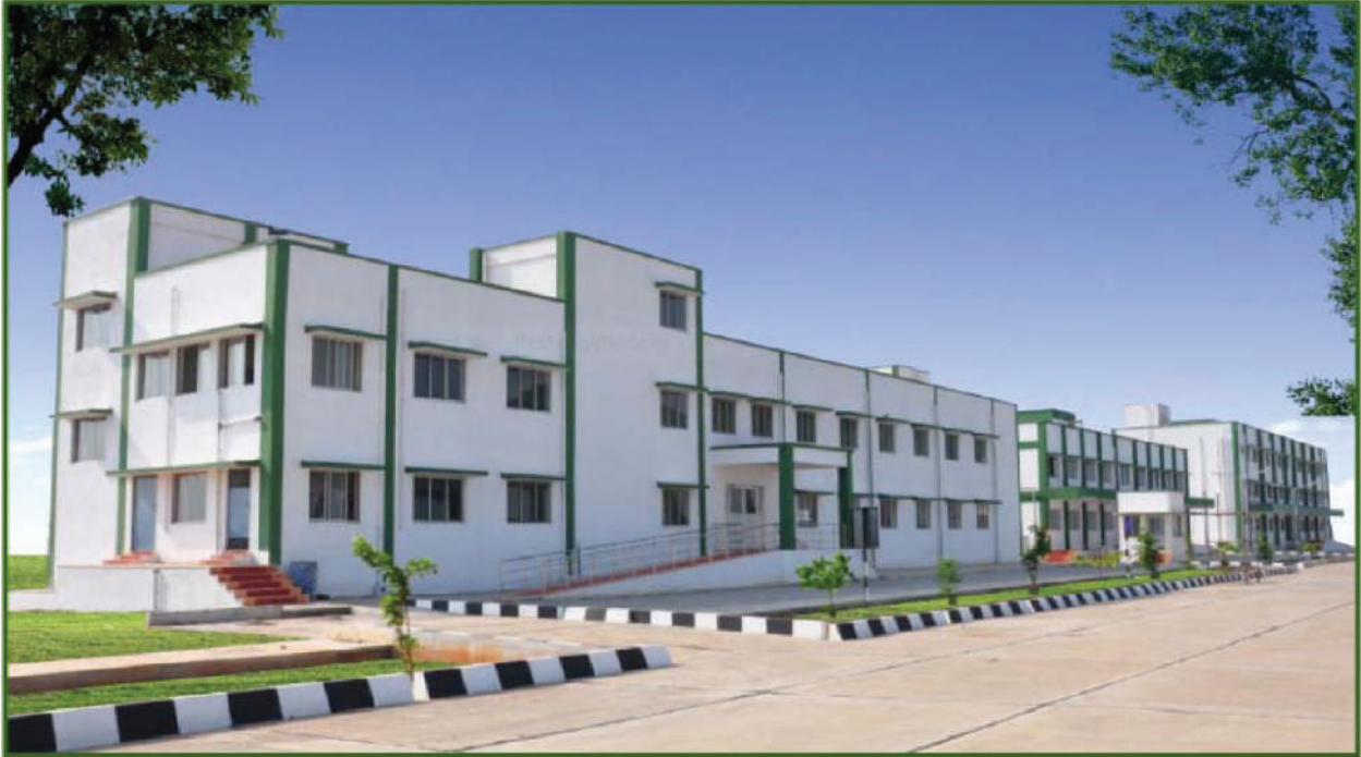
Modern Integrated Checkpost Incoming Office Building at Pethikuppam in Tiruvallur District
