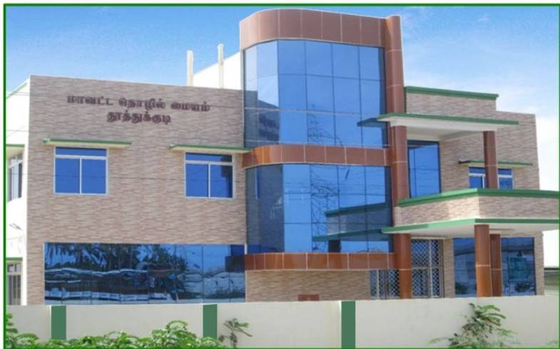
Additional building for District Industries Centre at Thoothukudi
