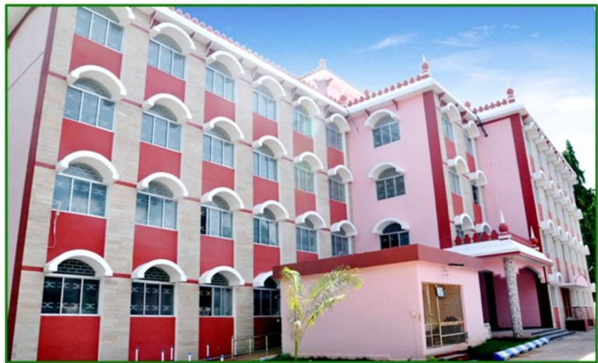
Combined Court building at Periyakulam in Theni District
