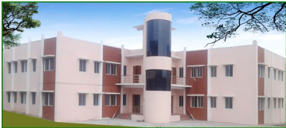
300 Nos Boys Hostel Building in Sainik School at Amaravathy Nagar in Tiruppur District under NABARD Scheme
