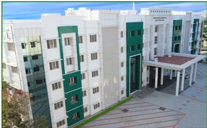
Multistoried Building for RCH Centre of Excellence in Government Mohan Kumaramangalam Medical College Hospital at Salem
