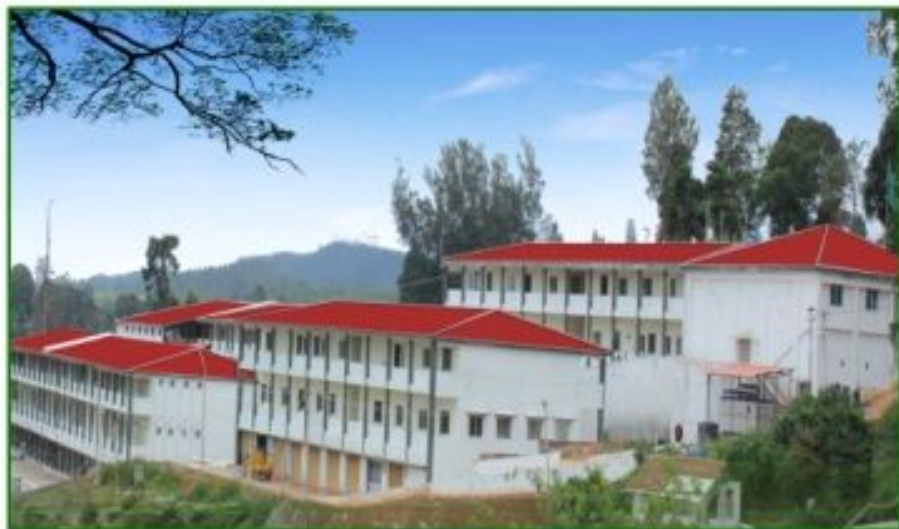
Additional Collectorate Building at Udhagamandalam
