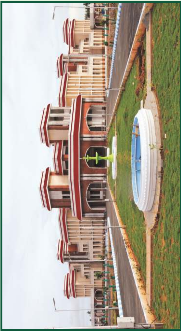
Collectorate Building at Cuddalore in Cuddalore District Rs.25.00 crore – Completed
