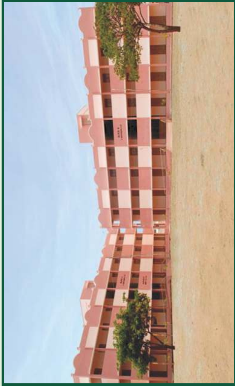
School Building at Mohanur in Namkkal District - Rs. 2.18 crore - Completed
