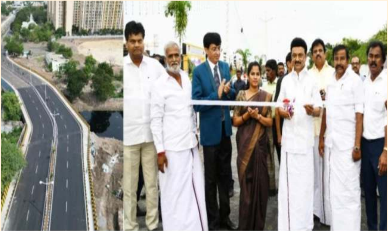
The Chengai Sivam Bridge in Stephenson Road (Thiru vi ka Nagar zone), constructed at a cost of Rs.66.83 Crore was inaugurated by the Hon'ble Chief Minister of Tamilnadu Thiru. M. K Stalin on 1.07.2023.
