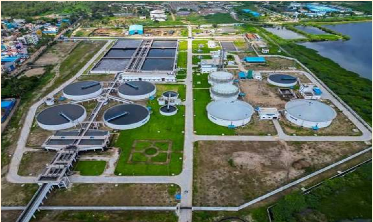
120 MLD (Zone - 2) Sewage treatment plant at Kodungaiyur.
