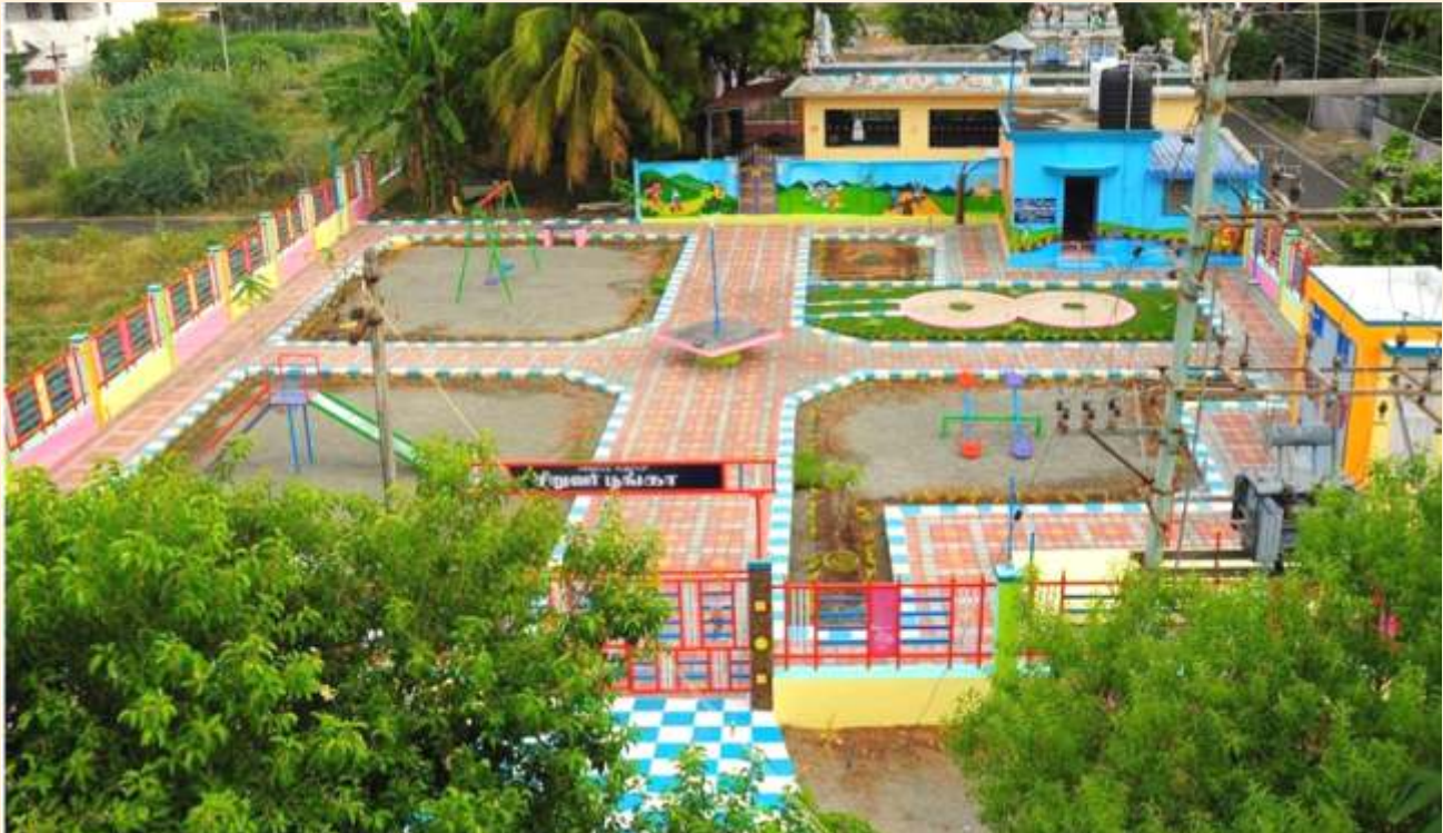
Improvement works to Childrens Park and Play Fields at Indira Nagar Park in Lakkampatti Town Panchayat, Erode District. Scheme Name: AMRUT 2.0, Estimate Cost Rs.26.50 Lakhs.
