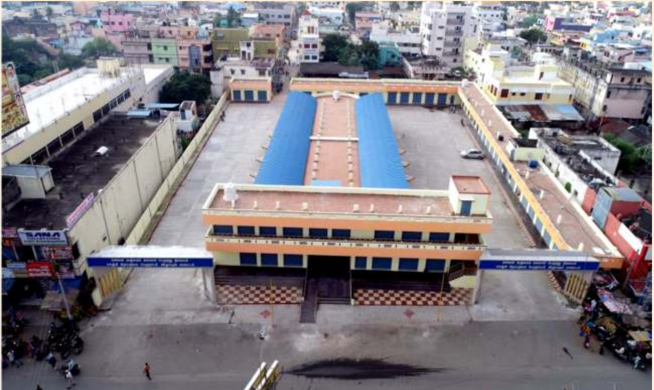
Construction of Bus Stand in Gingee Town Panchayat, Villupuram district, Scheme Name: KNMT, Estimate Cost - Rs.6.74. Crore
