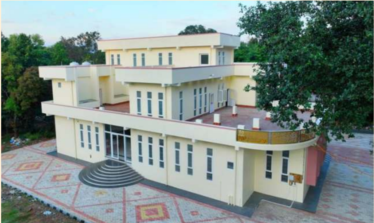
Construction of Knowledge and Study centre in Nagercoil Corporation. Scheme: Capital Grant Fund, Project Cost: Rs. 2.50 Crore
