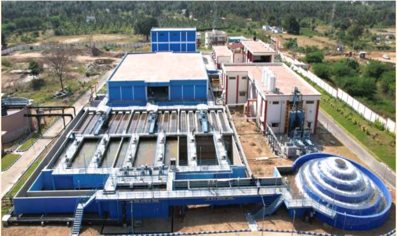
Water Supply Improvement Scheme to expanded Coimbatore Corporation with River Bhavani as source, Pillur-III. Water Treatment Plant- Thandiperumalpuram.
