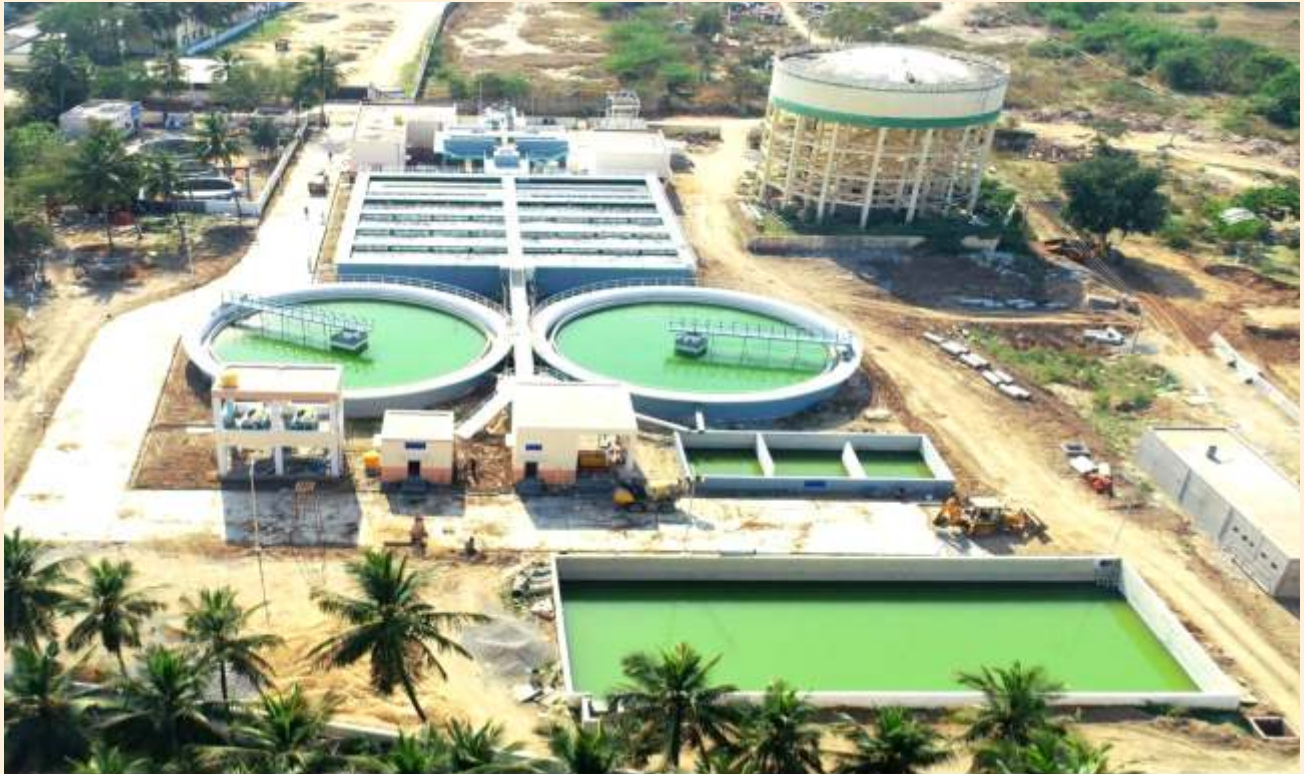
Underground Sewerage Scheme to Ambur Municipality in Tirupattur District - Sewage Treatment Plant - 16.71 MLD capacity at Kaspa.A - Ambur Municipality
