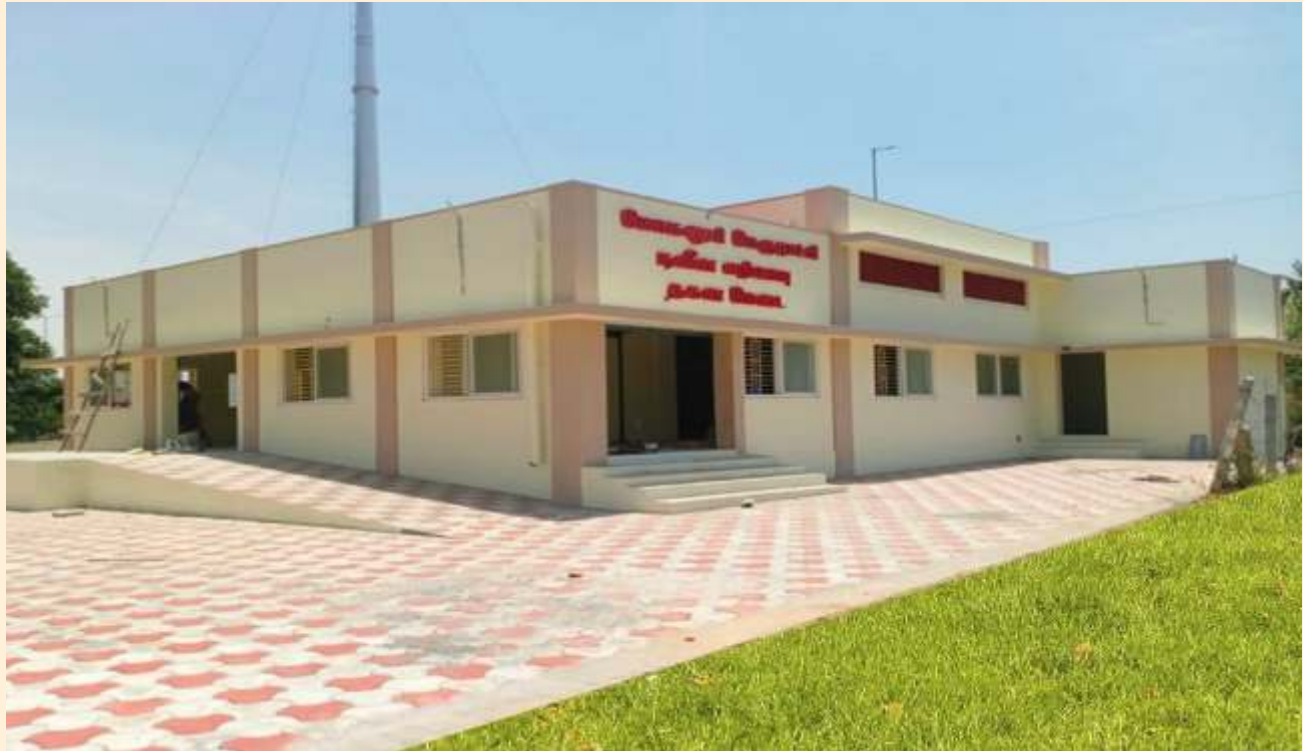
Namakkal District - Mohanur Town Panchayat. Construction Of Modern LPG Crematorium, Toilet Block and Parking Shed in Town Panchayat Burial Ground under KNMT, Estimate Cost: Rs. 1.50 Crore.
