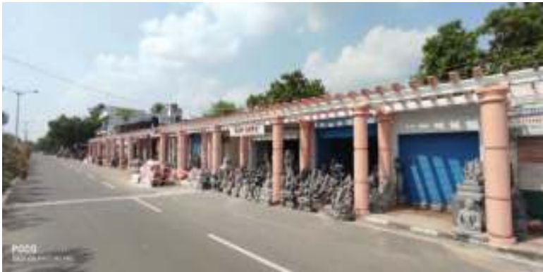
Beautification of Artisans work sheds at Five Rathas Street, Mamallapuram
