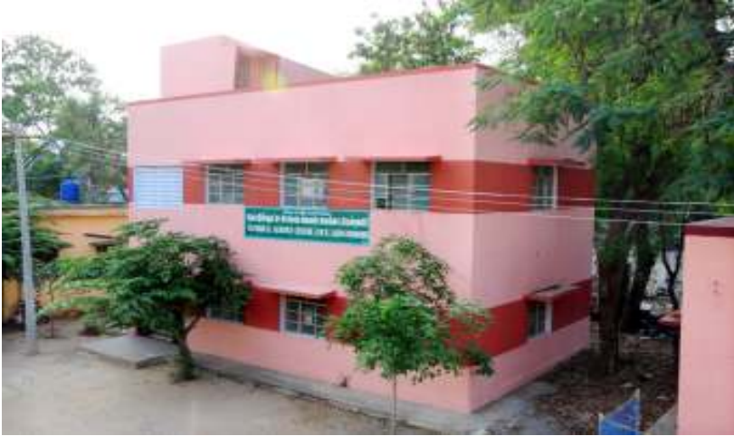
Technical Service Centre, Krishnagiri, Krishnagiri District
