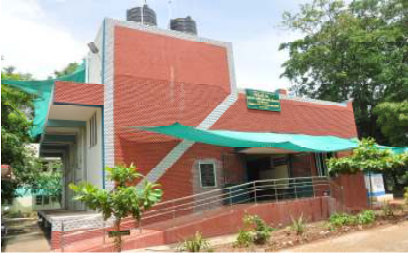
Multigraded Cold Storage Unit, Krishnagiri
