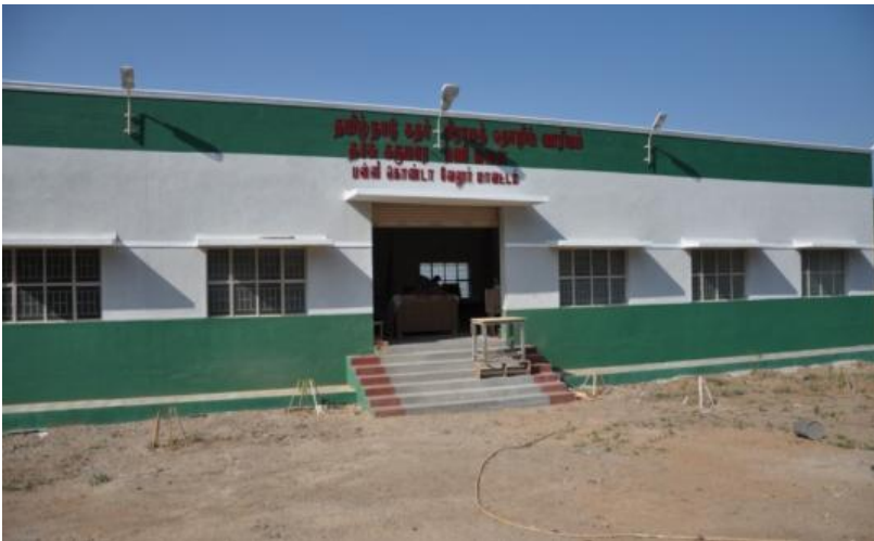
New workshed of Carpentry and Blacksmithy Unit - Pallikonda
