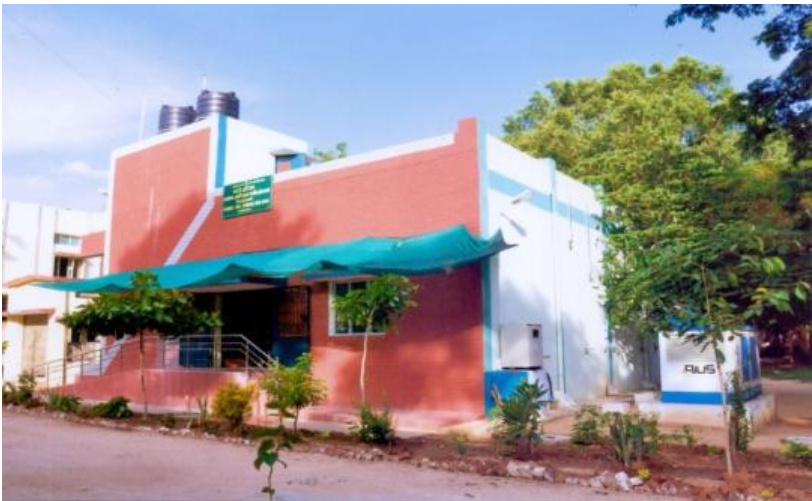
Multigraded Cold Storage Unit, Krishnagiri
