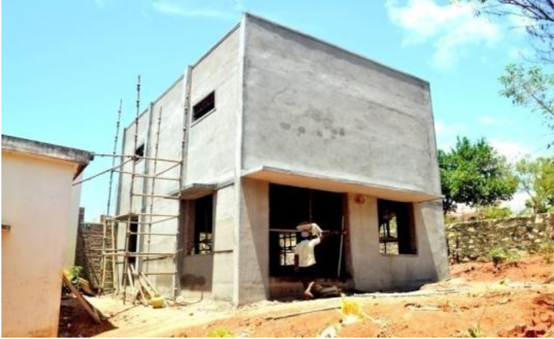
Construction of new building - Amsi
