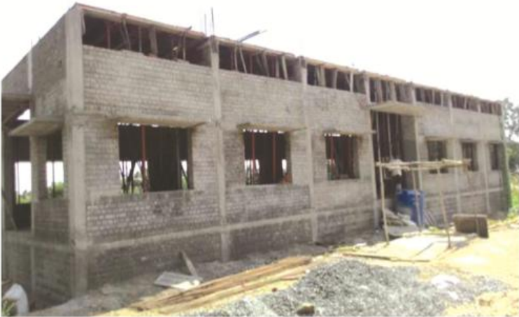
Work shed under Construction in Carpentry and Blacksmithy Unit at Pallikonda
