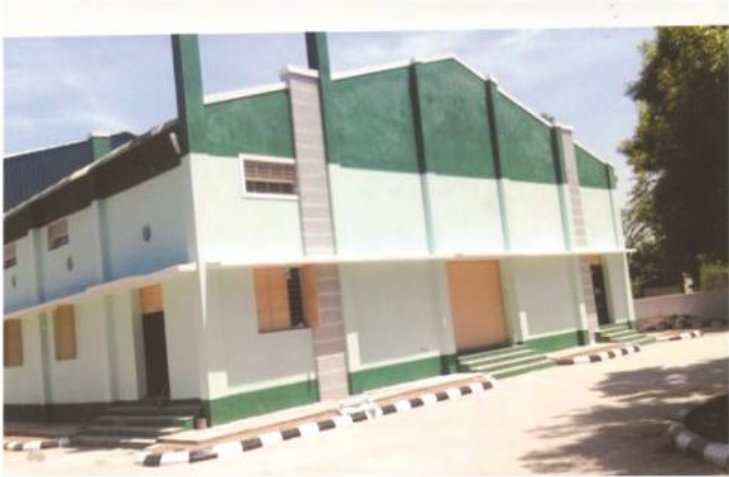
New building constructed for Automatic Bathing Soap Manufacturing Unit, Samayapuram
