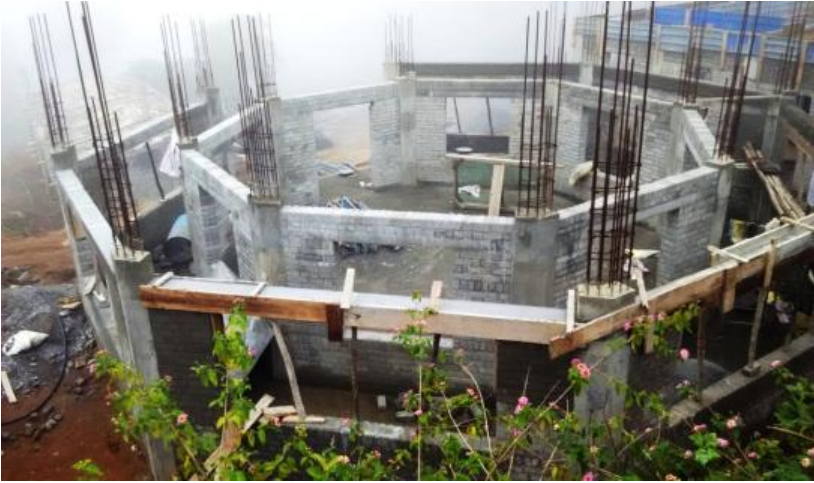
Construction of Children's Animation Centre
