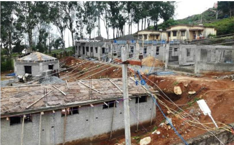
Construction of Sales Outlet
