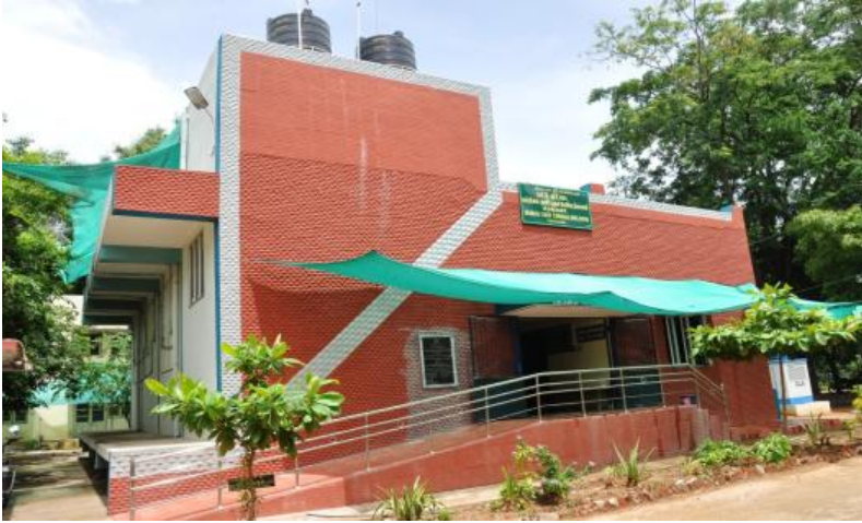
Hi-tech Cold Storage building at Bivoltine Grainage, Krishnagiri
