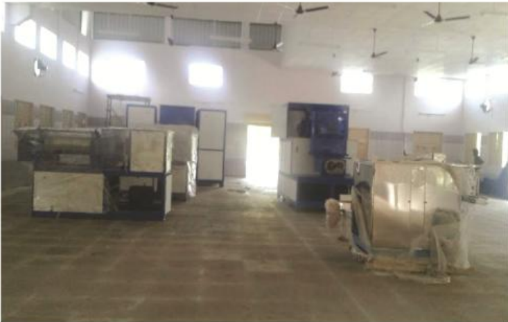
Automatic Bathing Soap Manufacturing Machine being installed at Samayapuram.
