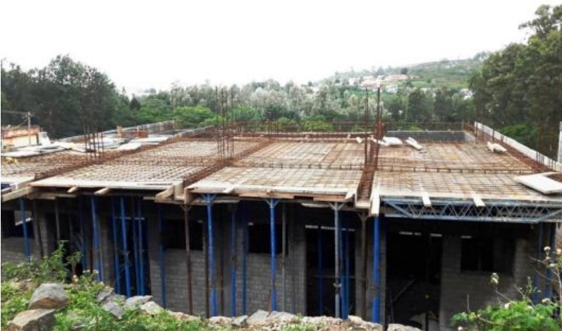
Construction of Food Court
