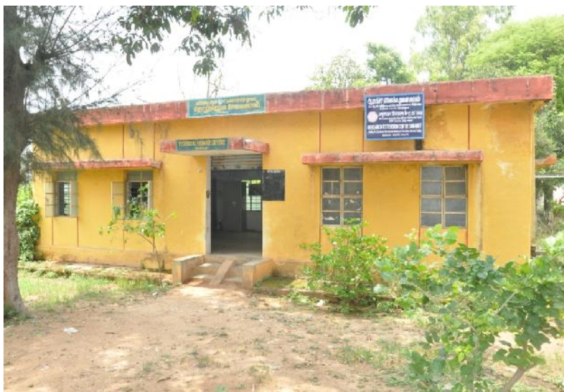
A Technical Service Centre at Berigai, Krishnagiri District
