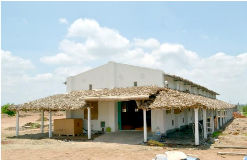
Rearing Shed constructed with Government assistance at a Mulberry garden in Dindigul District
