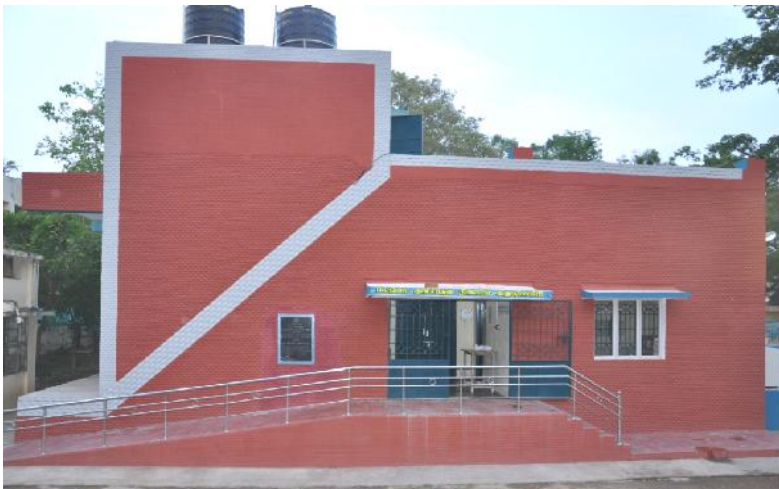
Recently Constructed Cold Storage building for Bivoltine Grainage at Krishnagiri
