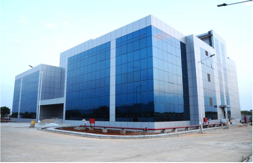
ELCOSEZ – Vadapalanji, Madurai
