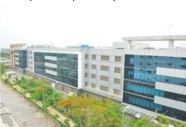
Figure-3 : M/s. TPCL, ELCOSEZ, Coimbatore
