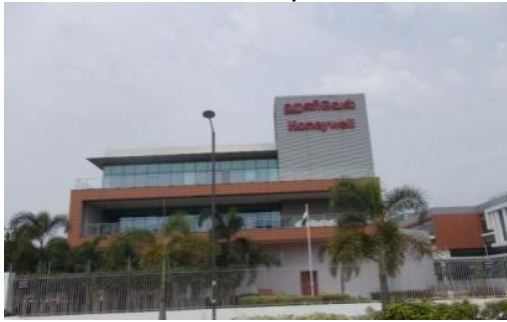
Figure-4 : M/s. Honeywell, ELCOSEZ Ilandhaikulam, Madurai
