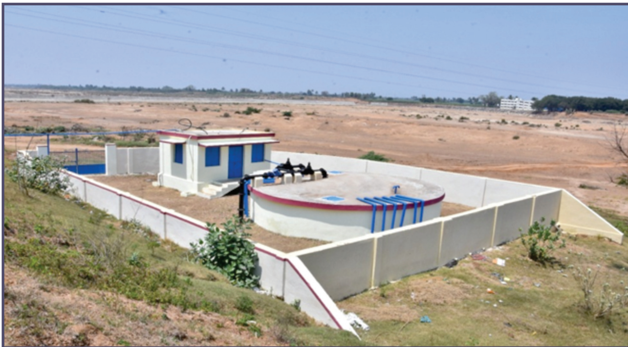
Combined Water Supply Scheme for 9 Panchayats in Panruti and Annagramam Unions of Cuddalore Districts at the cost of Rs.9.21 crore implemented from DMFT Fund
