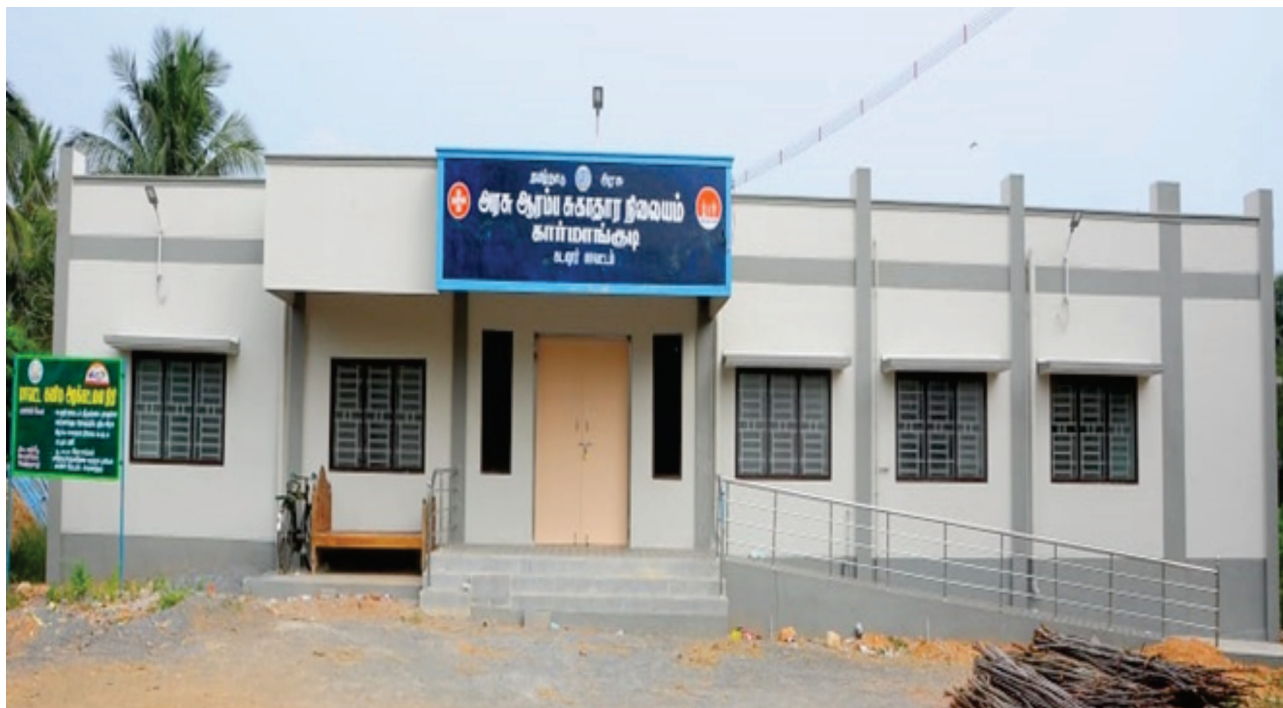
Construction of Primary Health Center at Karmangudi Village of Srimushnam Taluk in Cuddalore District at the cost of Rs.80 lakh
