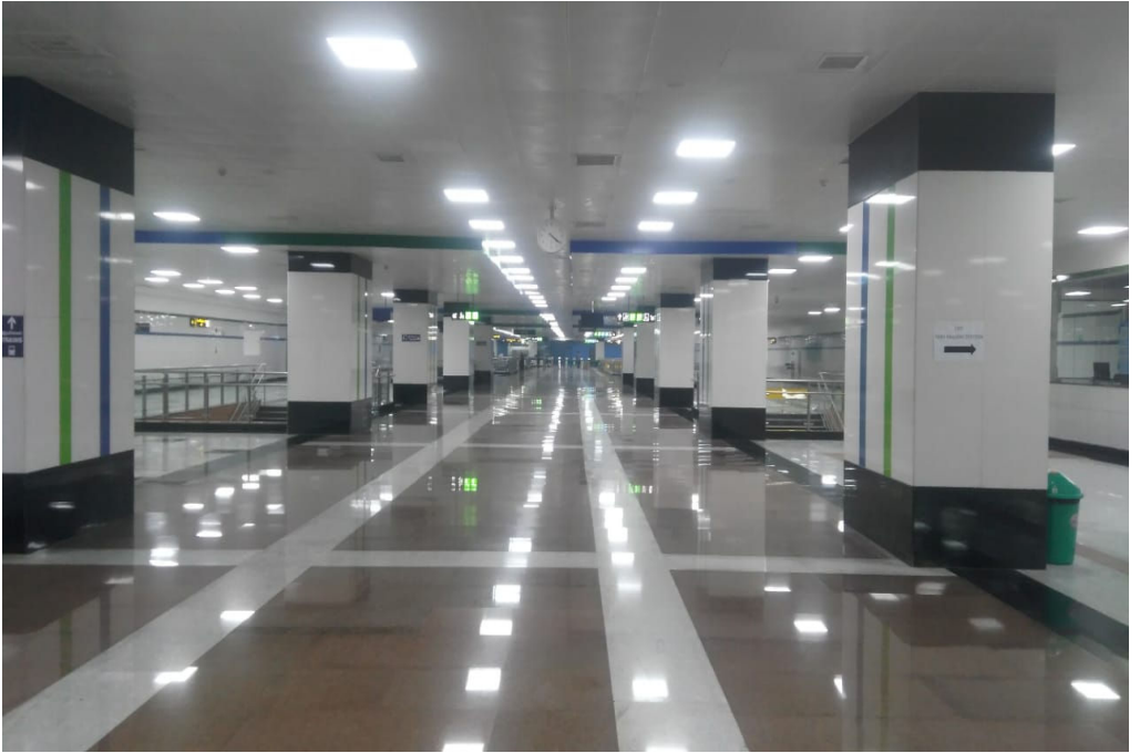
TAMIN – Granite flooring work done by TAMIN in Chennai Central Metro Station
