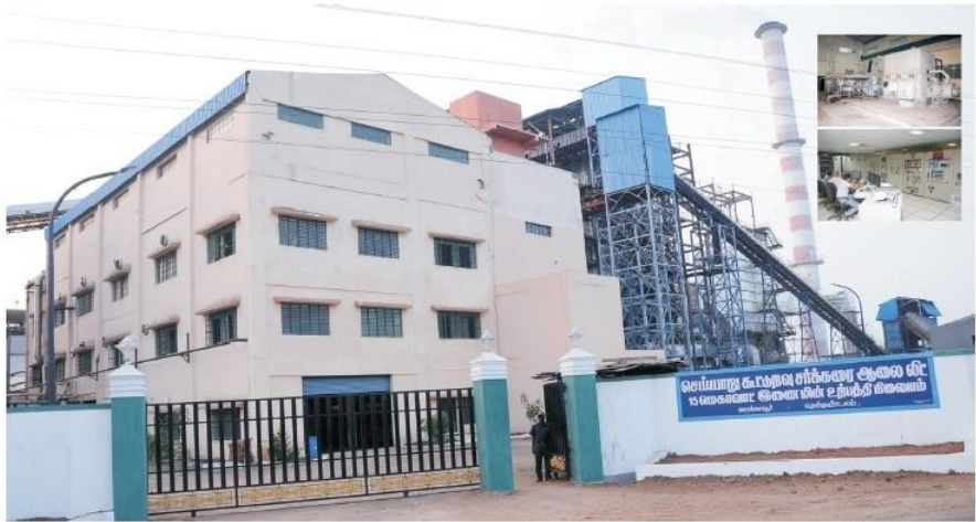
15 MW Co-generation Plant at Cheyyar Co-operative Sugar Mill
