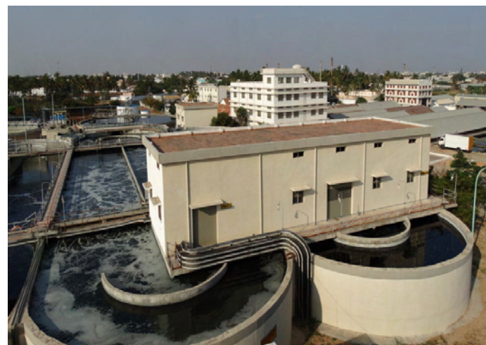
Common Effluent Treatment Plant
