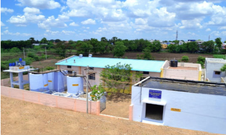
District Level Dye house with ETP facility at Arupukottai, Virudhunagar District under Virudhunagar Mega Handloom Cluster
