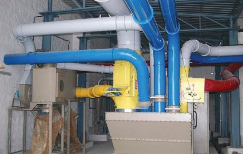
Automatic Washer Evacuation System at Ramanathapuram District Co-operative Spinning Mills
