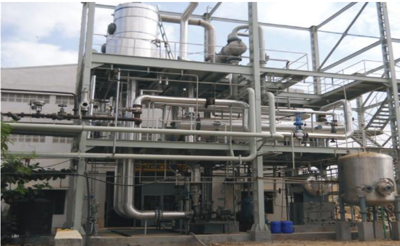
Mechanical Evaporator of Veerapandi CETP
