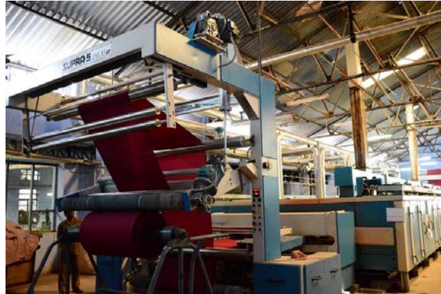
New Stenter Machine Installed at Tamilnadu Co-operative Textile Processing Mills Ltd., Erode
