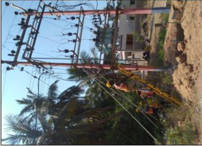
Replacement of Distribution transformers in Cuddalore
