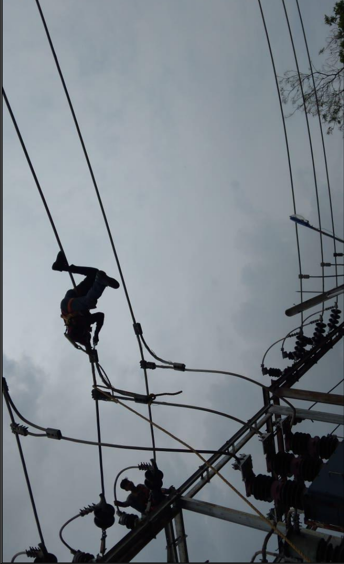
Damages Caused to Infrastructure due to GAJA Cyclone
