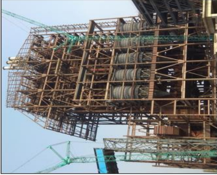
Electro Static Precipitator (ESP) and Boiler Works
