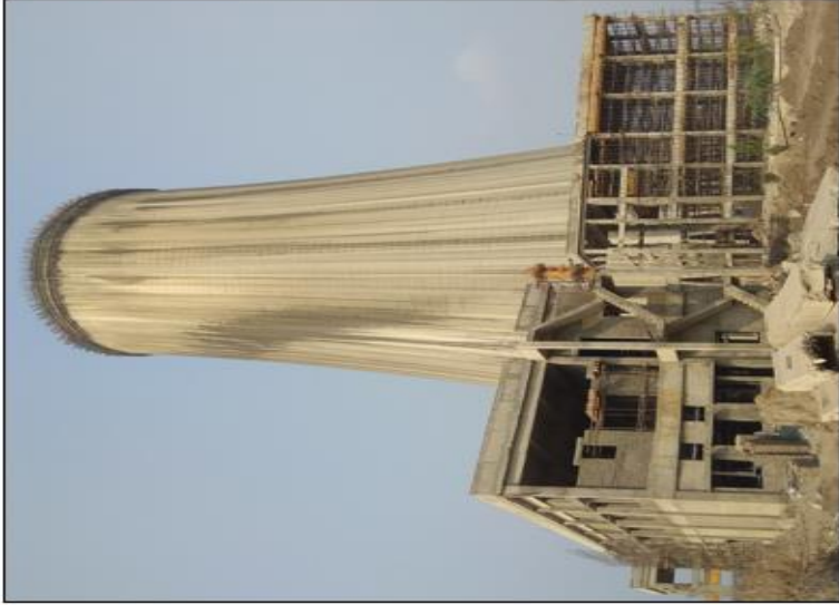
Natural Draught Cooling Tower construction Works
