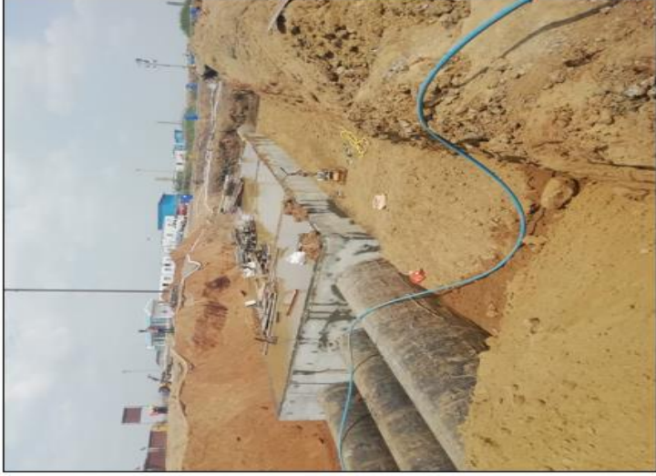
Fabrication of pipes in the Sea Water Intake & Out Fall System area
