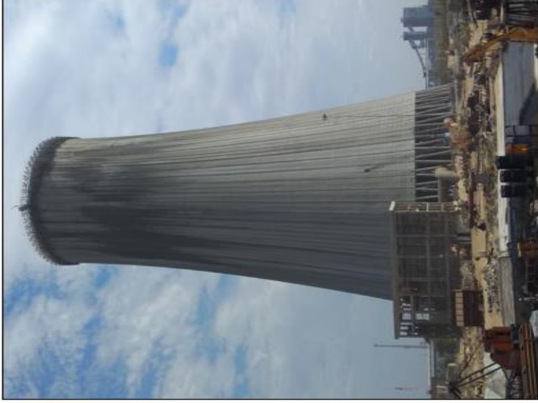
Natural Draught Cooling Tower construction Works
