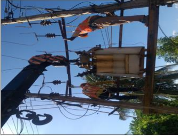
Replacement of Distribution transformers in Cuddalore
