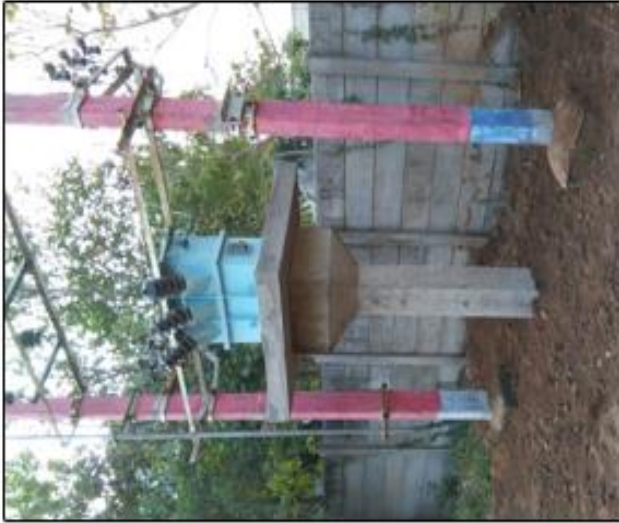
Replacement of Distribution transformers in Cuddalore
