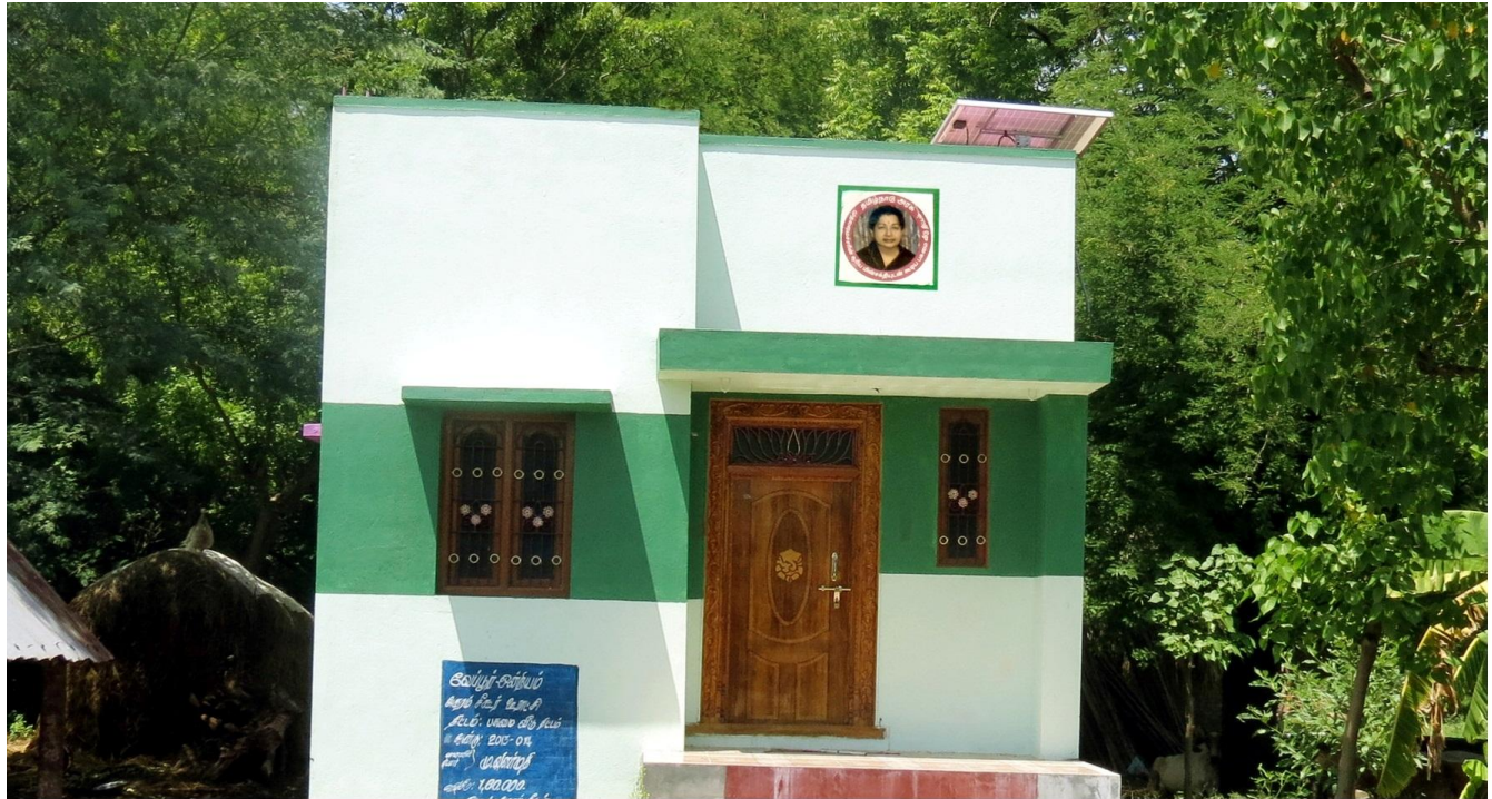
Hon'ble Chief Minister's Solar Powered Green House in Cuddalore District
