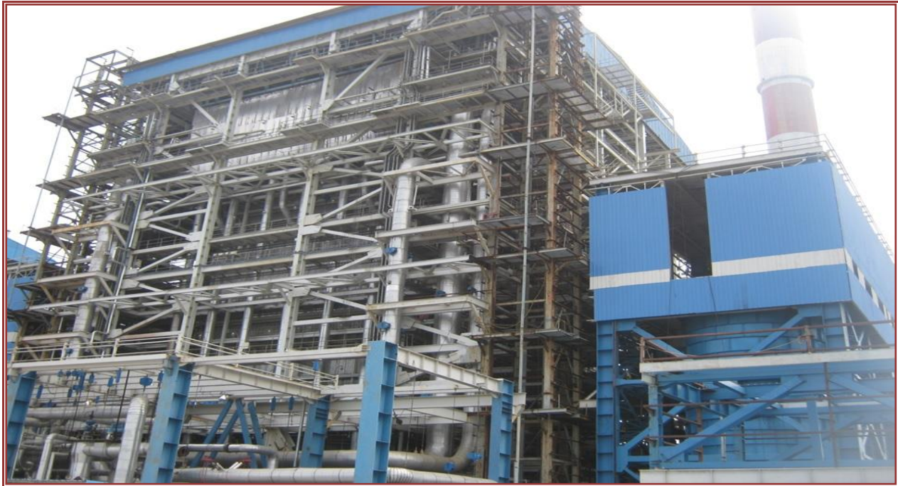
TANGEDCO-NTPC Joint Venture Project at Vallur, Unit 3 (3x500 MW)
