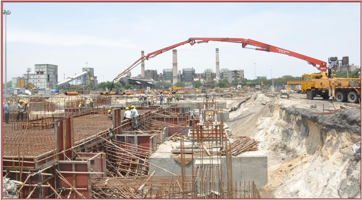
ETPS Expansion Thermal Power Project (1x660 MW)
