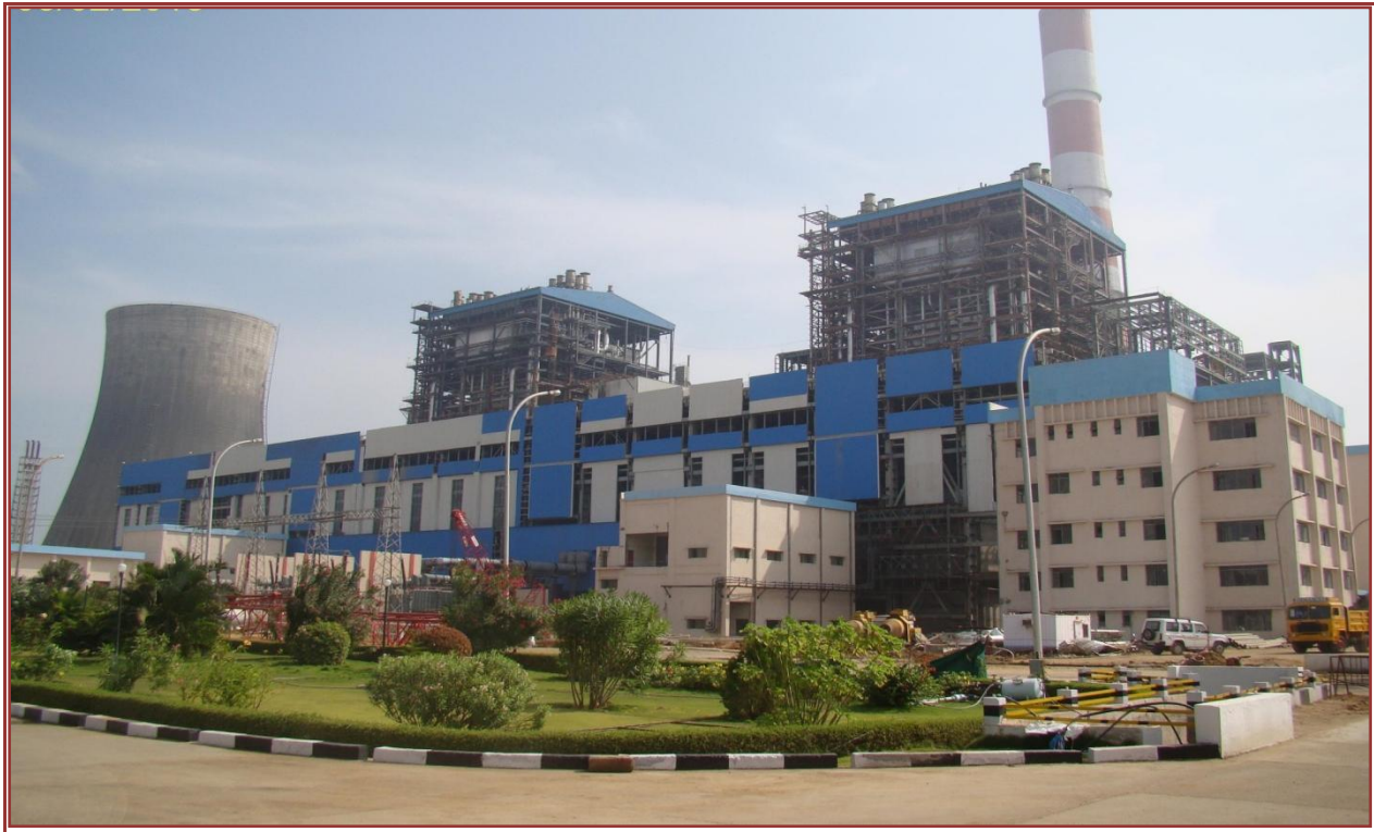
TANGEDCO-NLC JV Project at Tuticorin (2x500 MW)
