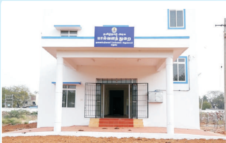
Madurai Deputy Registrar (Dairying) Building Inaugurated by Honourable Chief Minister on 13.03.2018
