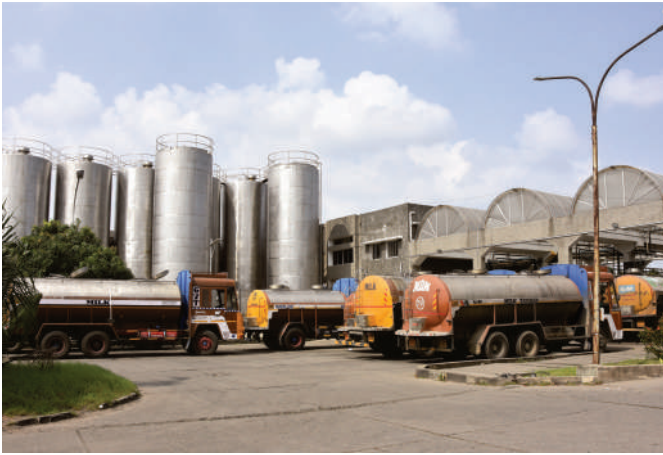
Milk Storage Silos
