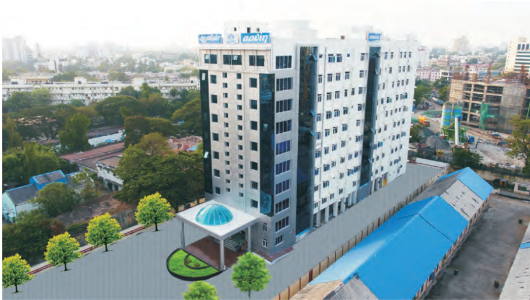
New integrated Aavin Administrative Building at Nandhanam
