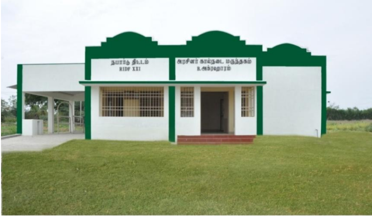
Veterinary Dispensary at P.Agraharam, Dharmapuri district constructed under NABARD RIDF XXI
