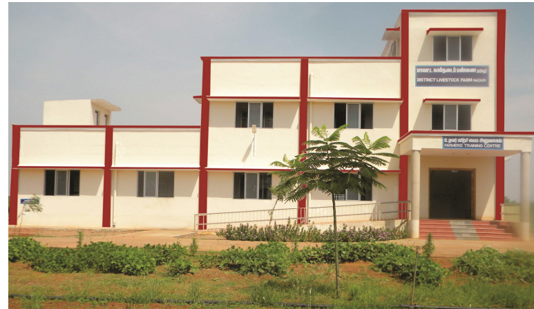
Farmers Training Centre at District Livestock Farm, Naduvur, Thanjavur district constructed under NADP
