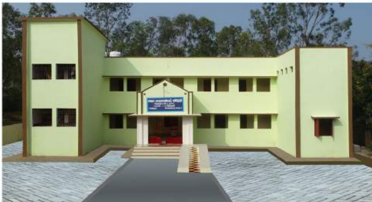
The newly constructed Adidravidar Welfare School Girls Hostel Building at Pounjur in Chengalpeta District (Estimate Amount: Rs. 111.03 Lakh).
