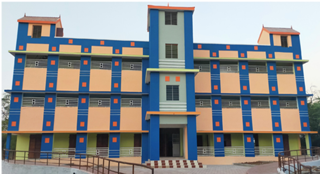
Newly constructed 12 classroom building in Nallammalpuram Adi Dravidar Higher Secondary School, Tirunelveli District.
