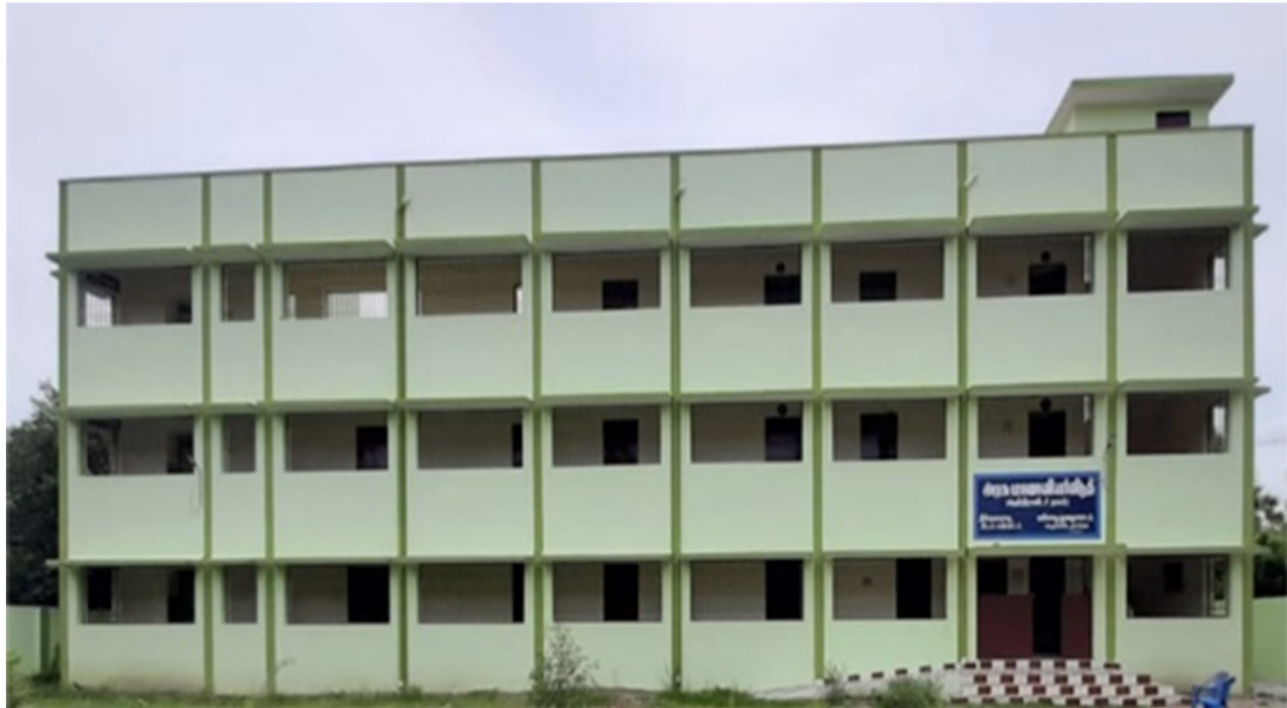
Hostel Building for Girls students of Adi Dravidar Welfare school in Thillaiyadi, Mayiladuthurai District
