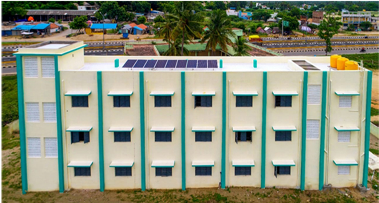
Hostel building for the students of Polytechnic college in Krishnagiri, Krishnagiri District.
