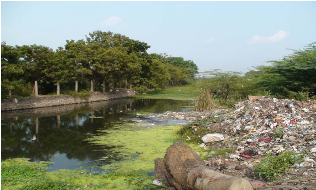
Solid Waste disposal in river
