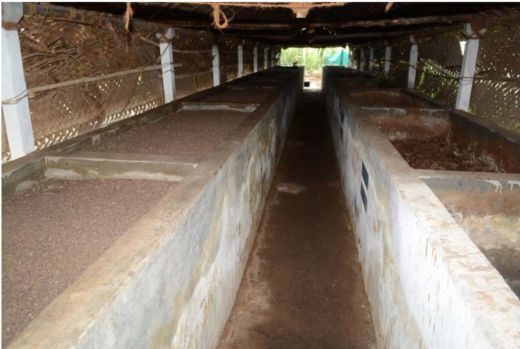
Vermi compost yard at Thudiyalur Town Panchayat.
