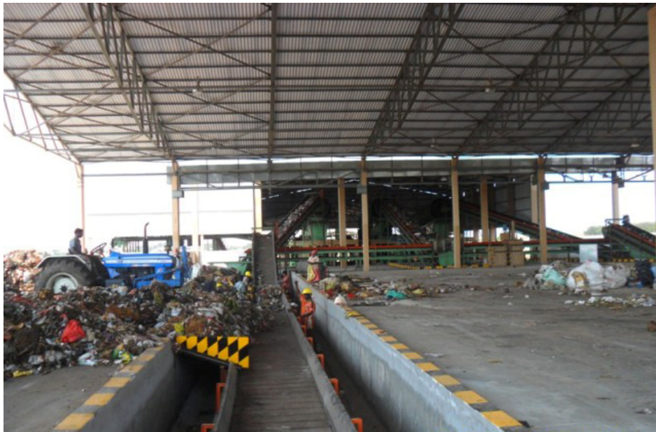
Integrated modern solid wastes transfer station at Peelamedu, Coimbatore.
