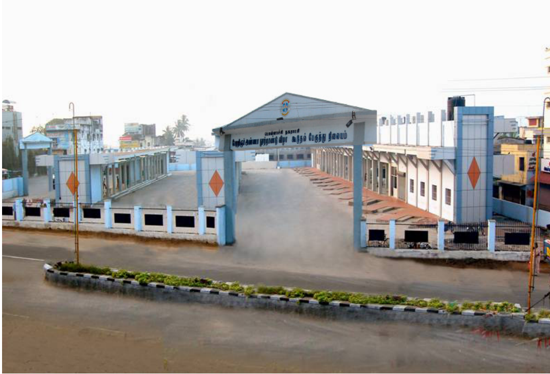
New bus stand constructed by Pollachi Municipality from own funds and loan.
