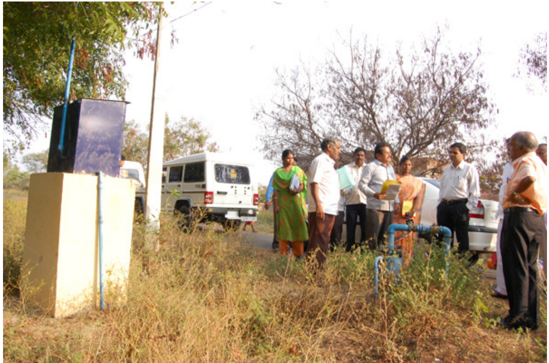
Deep bore well installed at Thaniyamangalam, Melur block, Madurai District through remote sensing
