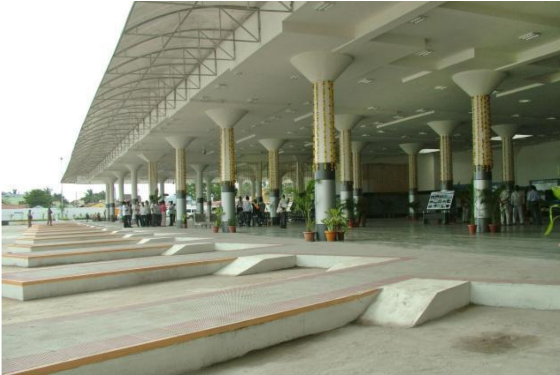
New bus stand constructed with modern facilities at Mettupalayam Road, Coimbatore
